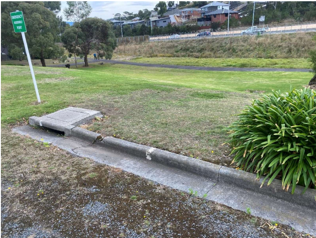
Figure 3 - Existing Kerb & Channel collecting carpark runoff, and the roadside overland flow path in background.
