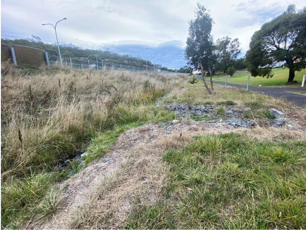
Figure 2 - Large table drain adjacent Rokeby Road, DN300 culvert under footpath to the right.
