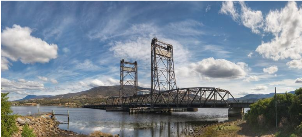
Figure 1-1: Photograph of Current Vertical Lift Bridge completed in 1946
