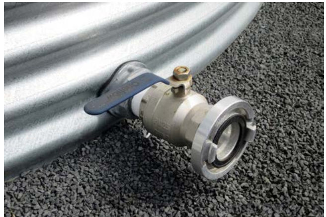
Figure 3 A water connection point with Storz coupling
