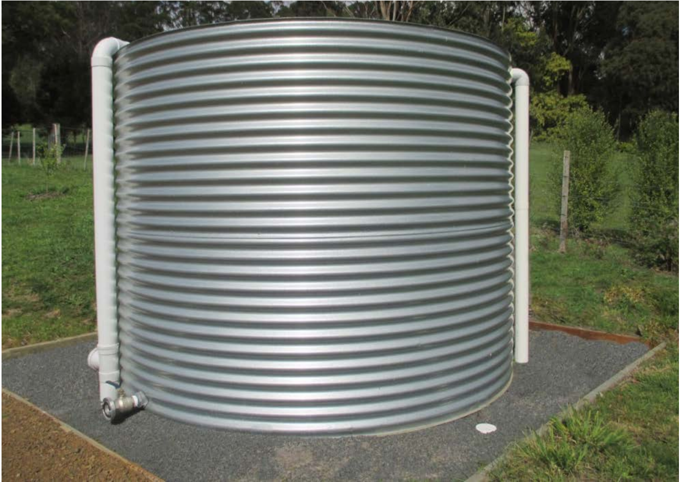
Figure 2 Compliant 10,000 litre firefighting water tank
