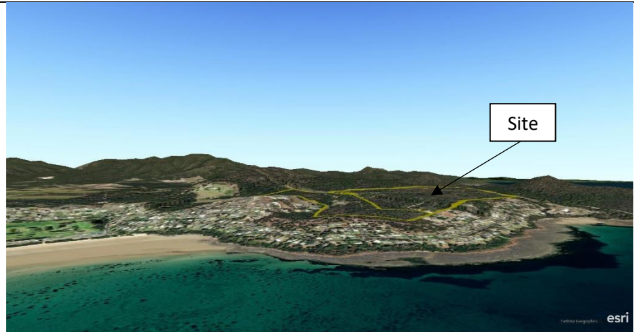
3D Image of the site contributing to the landscape setting of Greens Beach
