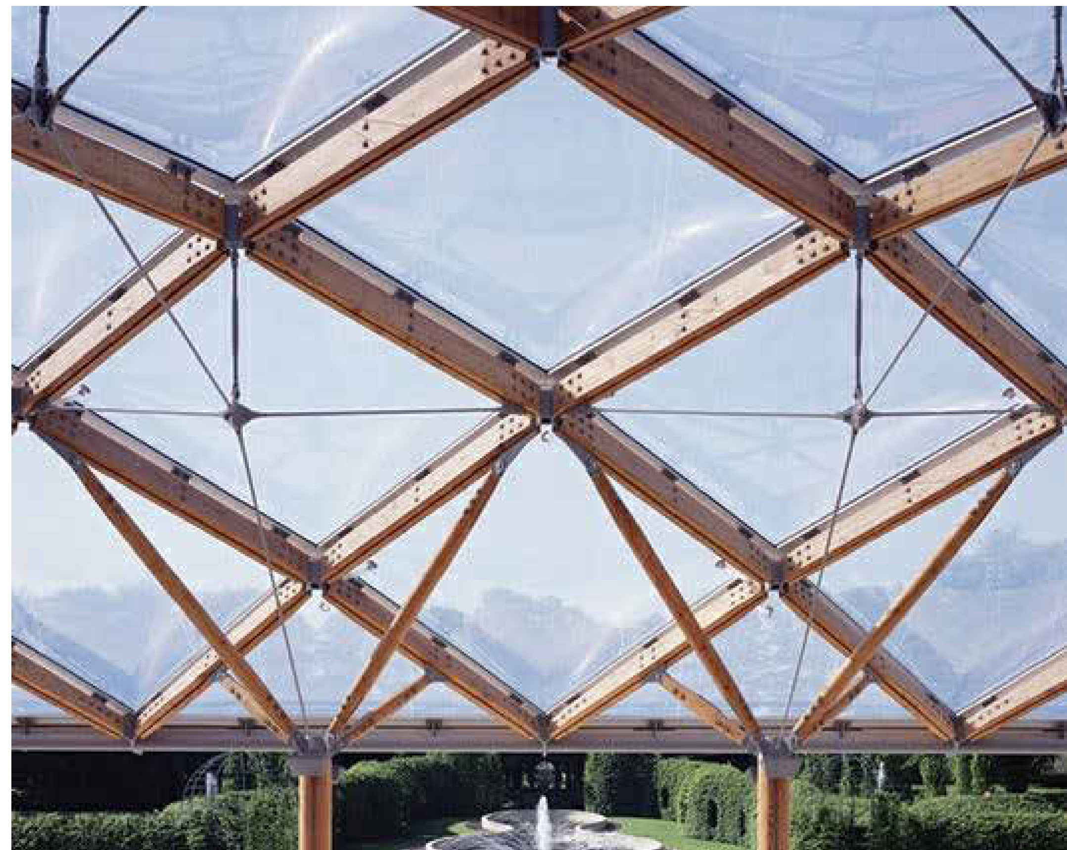
RT01 STEEL AND GLULAM HYBRID ROOF STRUCTURE WITH ETFE PILLOWS AND INTERGRATED GUTTER
