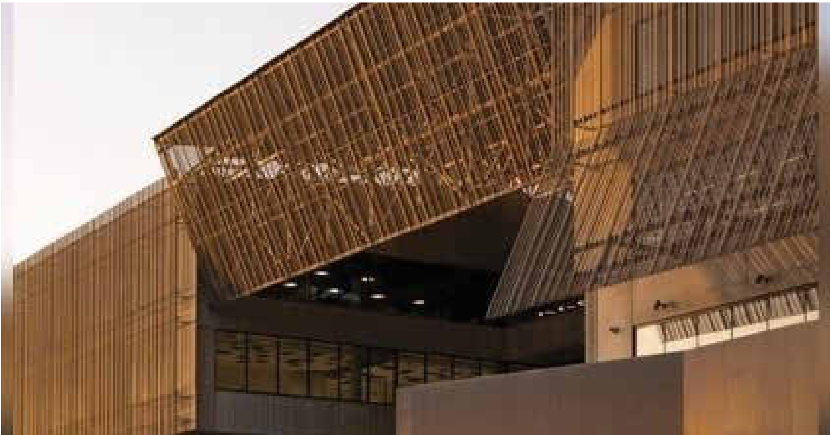
FT01 BATTEN SCREEN FIXED TO METAL CLADDING WITH GLAZED OPENINGS
