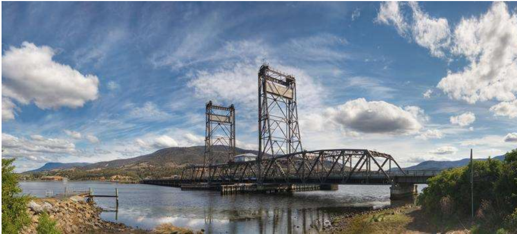
Figure 1 - Photograph of Current Vertical Lift Bridge completed in 1946
