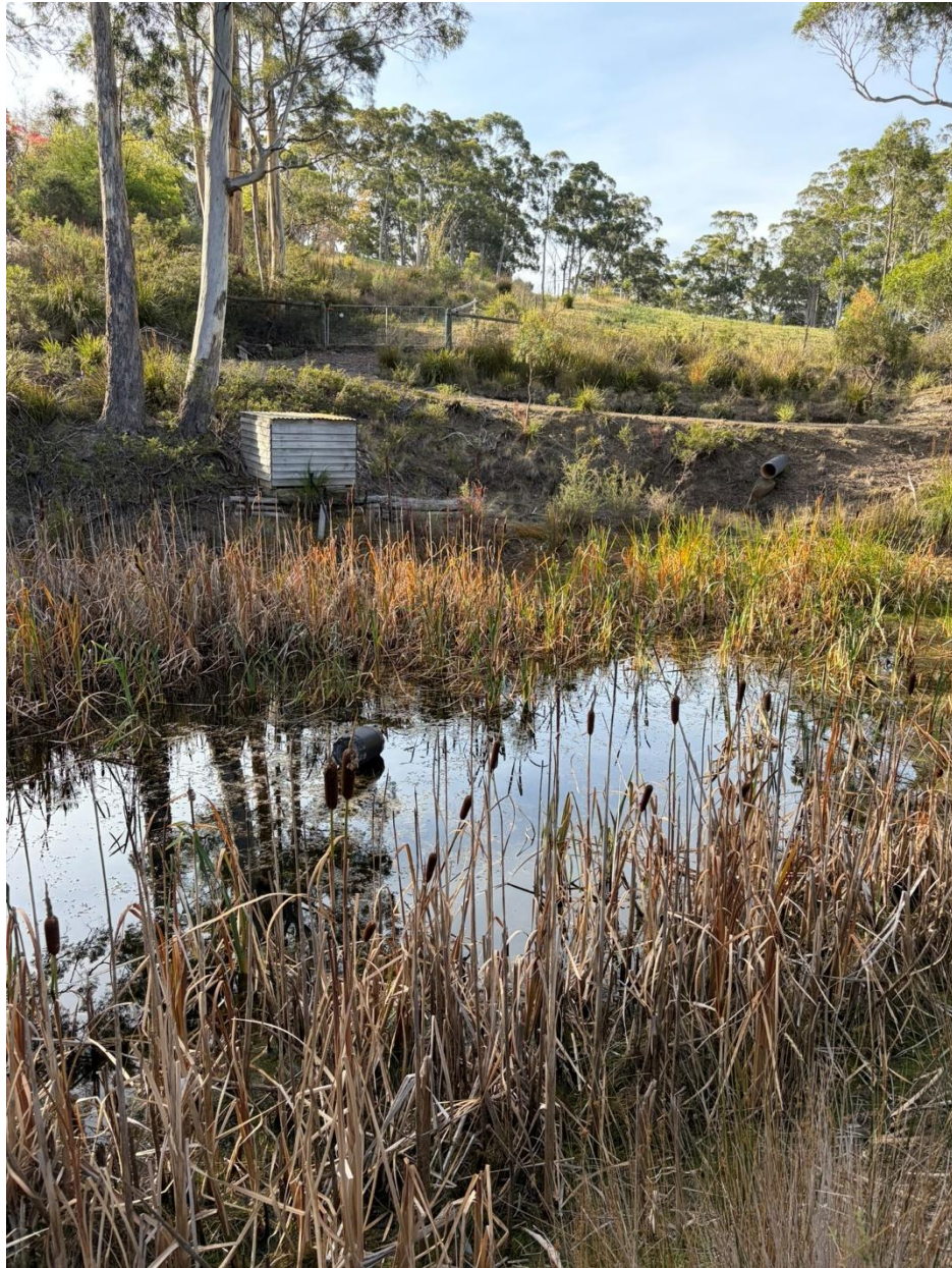
Figure 32: Irrigation and fire water dam (dam #5) and water management infrastructure.
