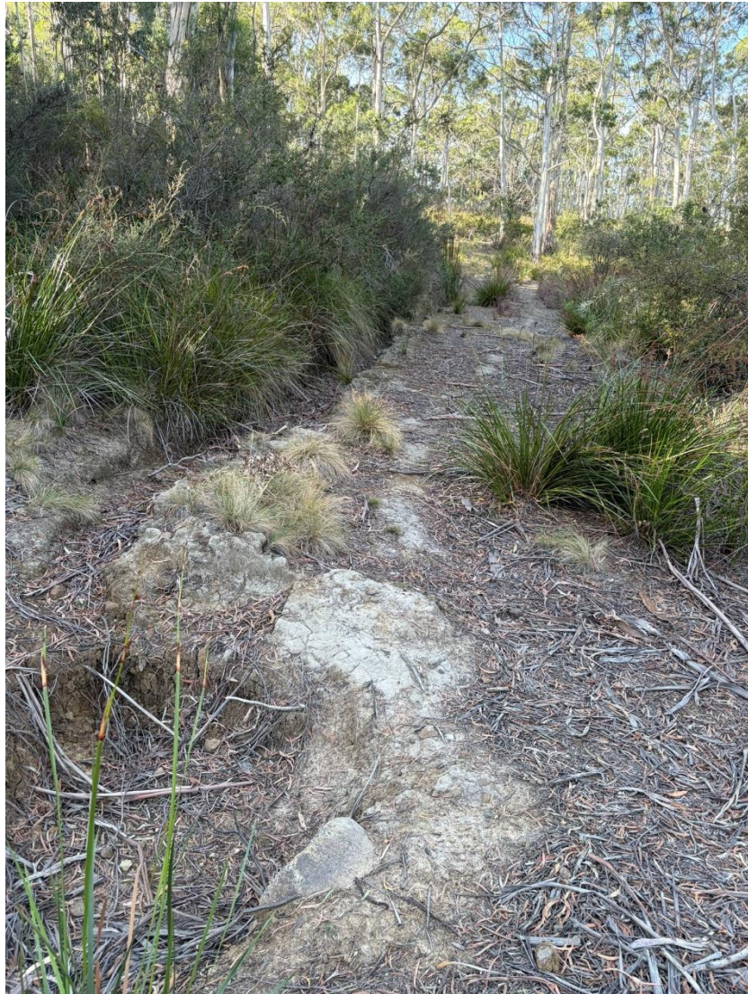
Figure 31: Water capture trench leading to culvert.
