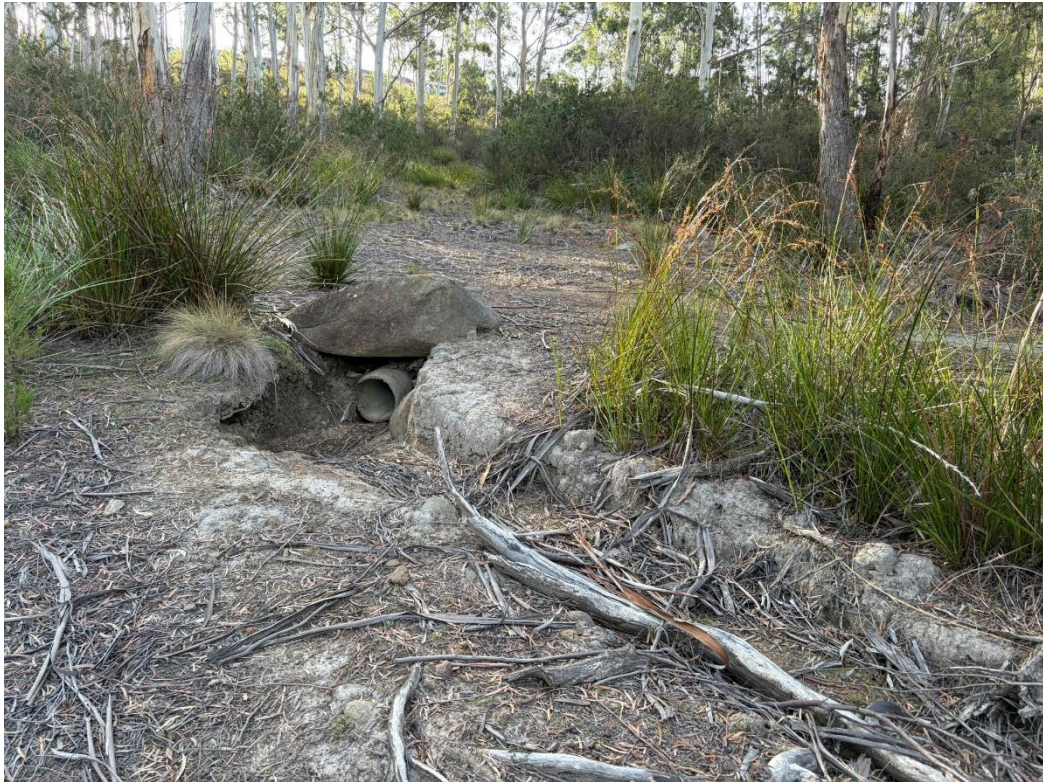
Figure 29: Water management development to capture water into dams.
