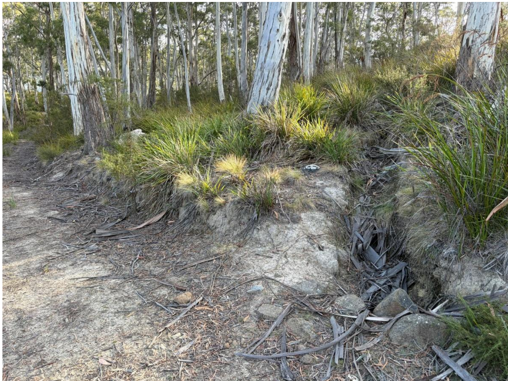
Figure 30: Example of trenching into culverts on right hand side, diverting water to dams.
