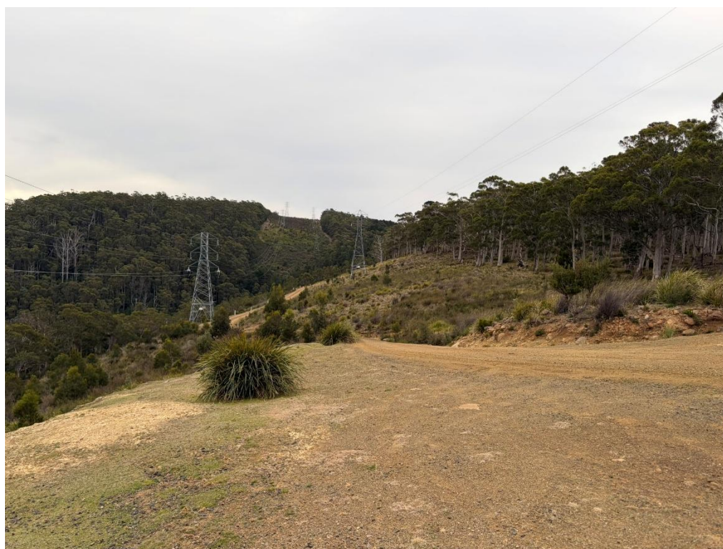
Figure 34: High voltage TasNetworks easement on the property.
