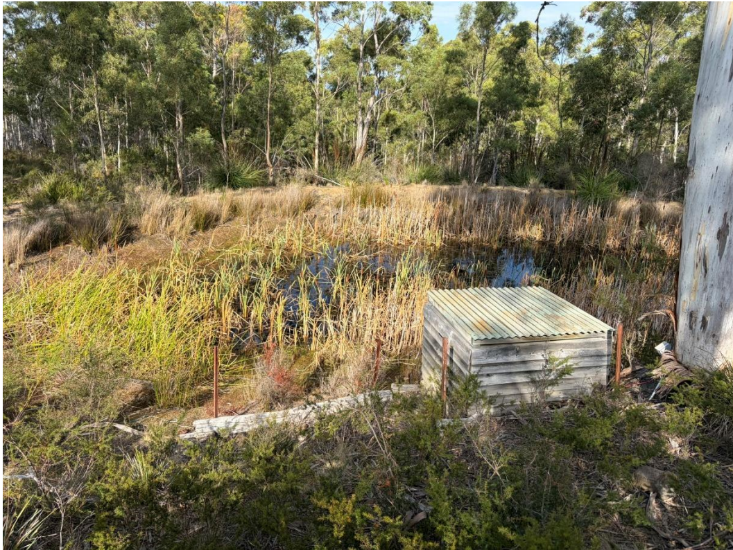
Figure 15: Irrigation and fire water dam and pump house.
