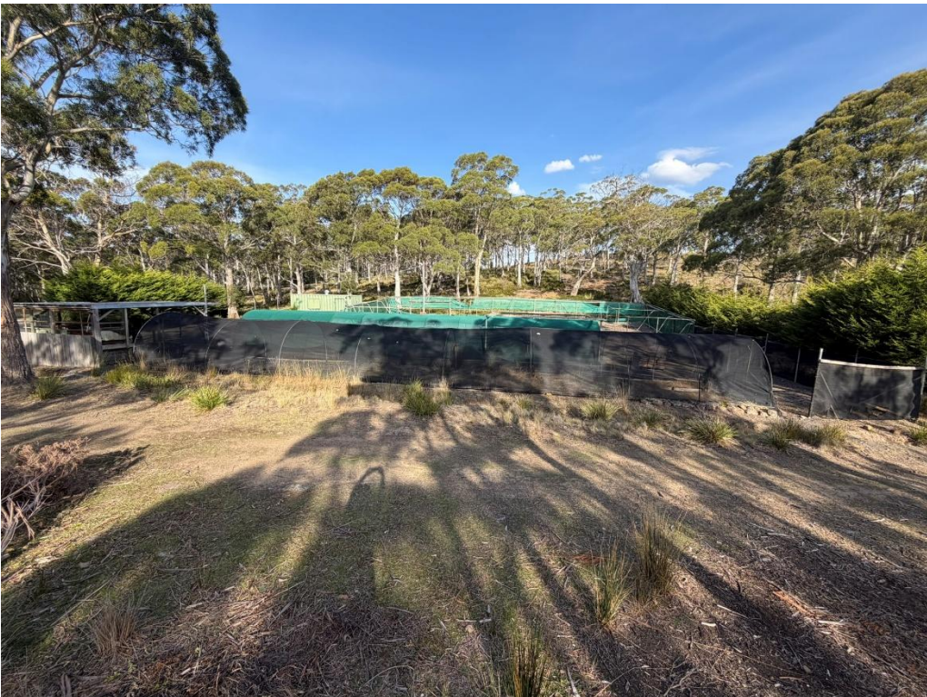
Figure 22: Old nursery infrastructure remaining onsite.
