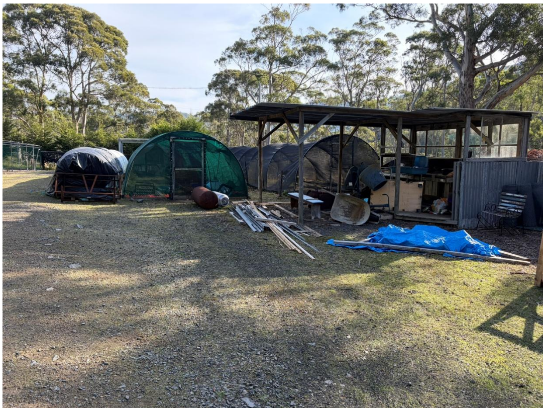
Figure 20: Old Nursery infrastructure remaining onsite.
