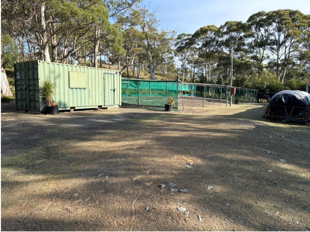
Figure 21: Old nursery infrastructure remaining onsite.
