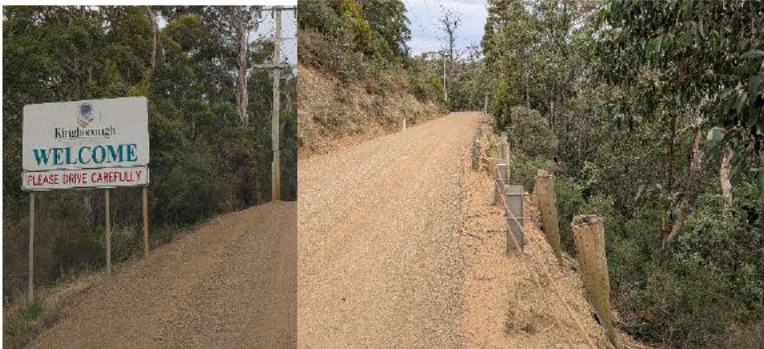
Figures 2-4. Summerleas Road, Fern Tree within Kingborough Council has retained much of its original character. Namely steep, tight curves on an irregular gravel surface. Recent installation of safety wire by the council has prevented most (but not all) vehicle traffic from falling off the edge of the road.
