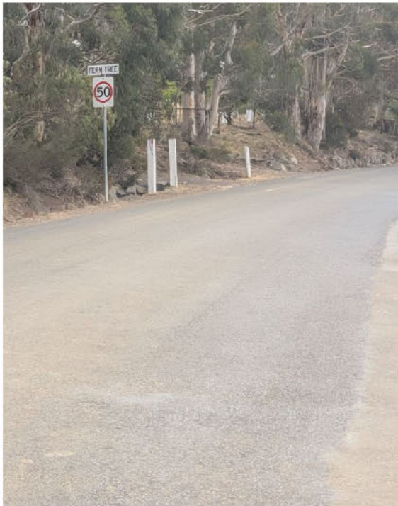
Figure 1. Summerleas Road, Fern Tree within Hobart Council has been upgraded to modern standards including bitumen
