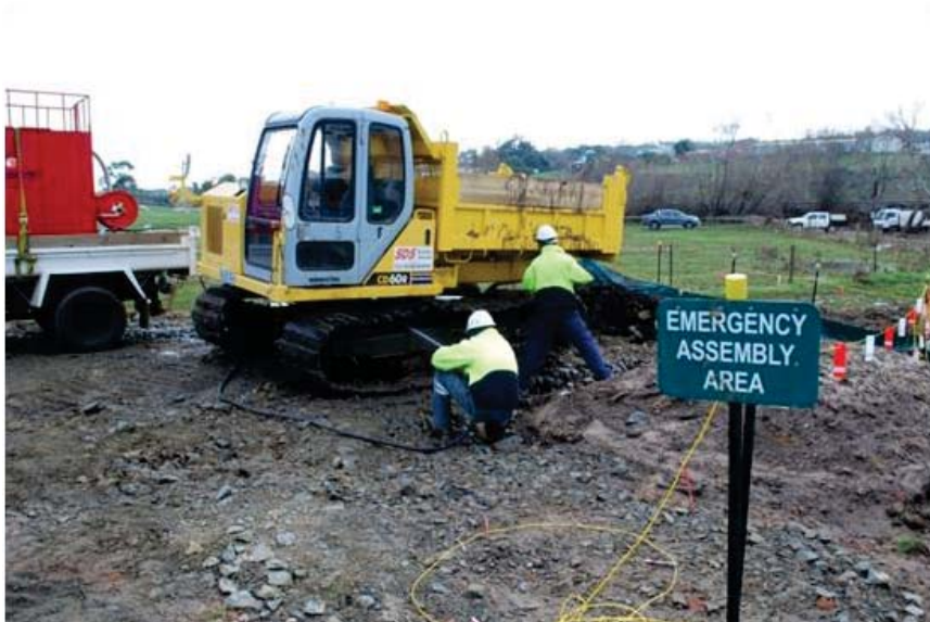
Temporary cleandown area
