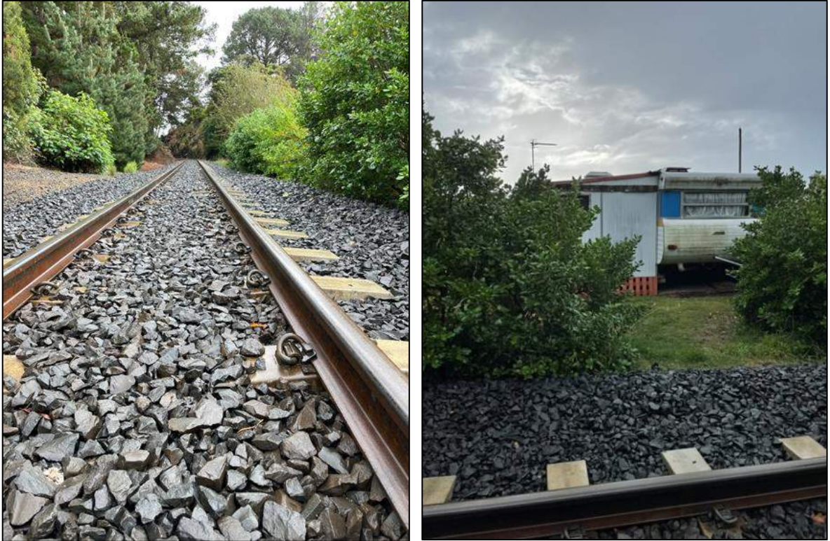
Figure 42: Western Line railway corridor (Source: I Duckett, 2021)
