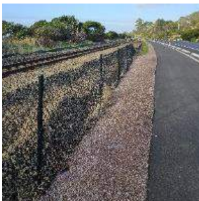
Figure 8: Permanent sturdy close cross mesh wire fence minimum 1200 mm high with 100 mm dug into the ground to prevent penguin access.
