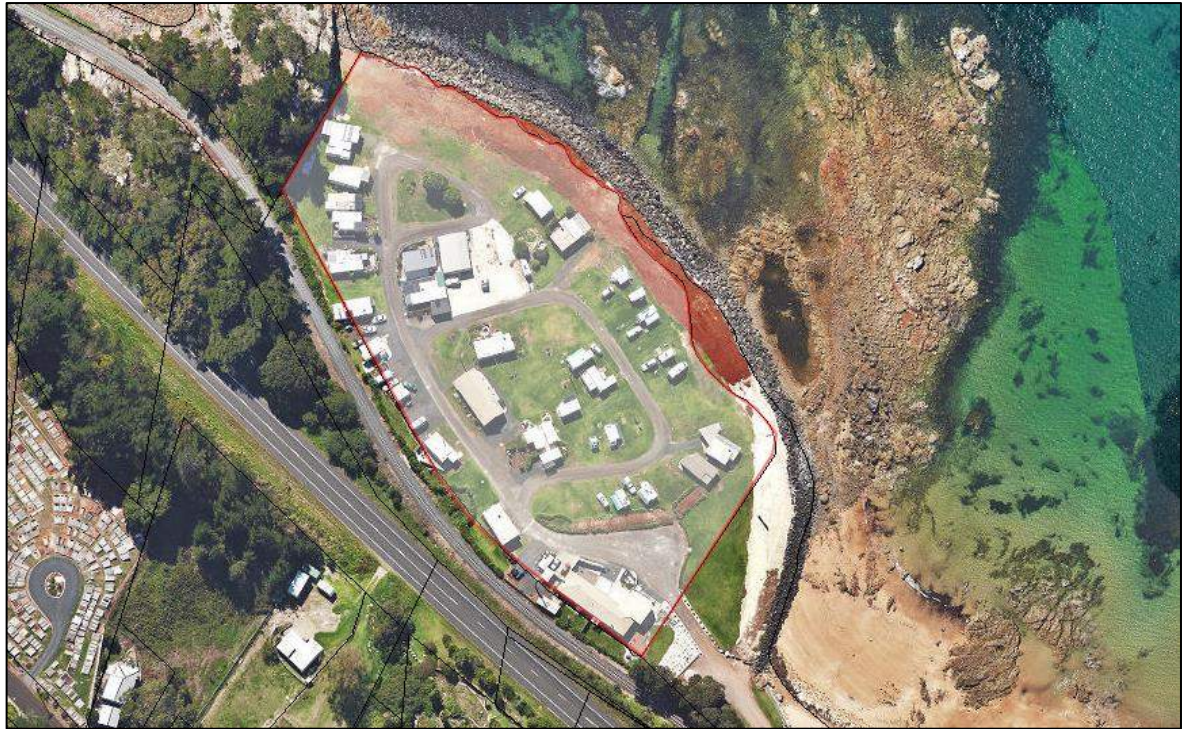
Figure 2: Aerial photo of existing structures on site (Source: www.theLIST.tas.com.au © State of Tasmania)
