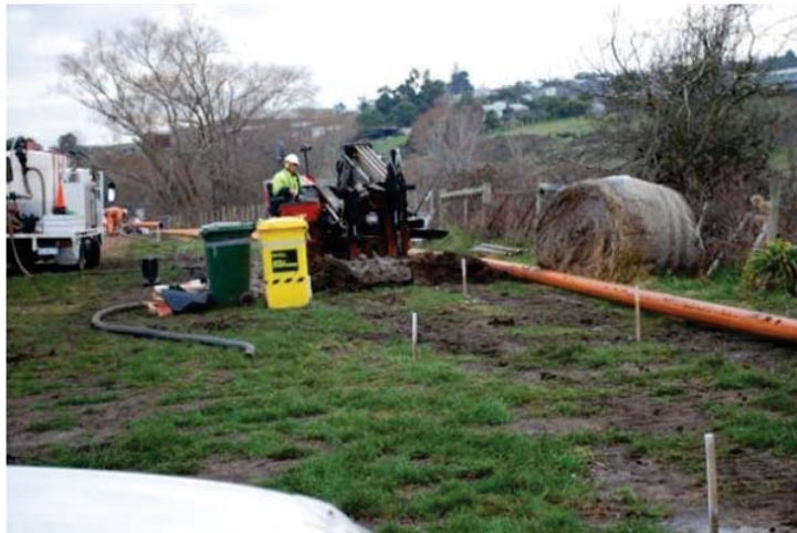
Cleaning down digging machinery
