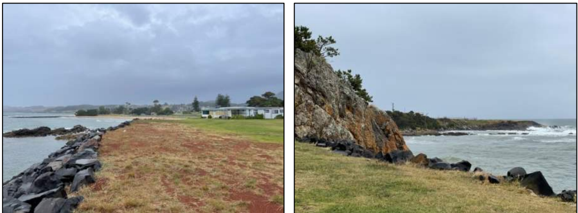
Figure 45: Images of coastal protection works (source I Duckett, 2021)
