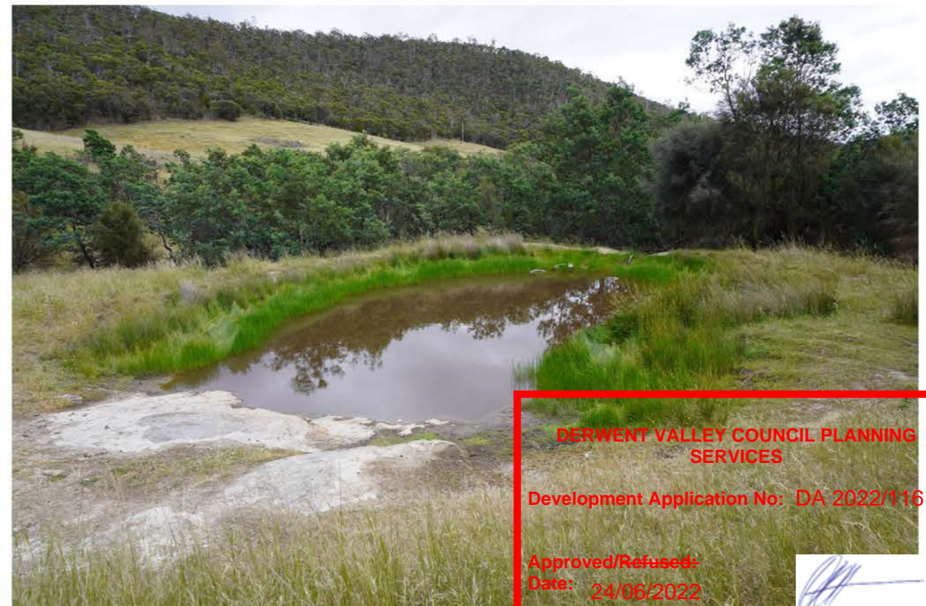
STORMWATER DETENTION POND PHOTO 9
