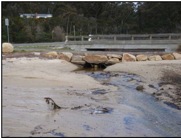
Figure 144.4. Restricted flow through pedestrian walkway.
