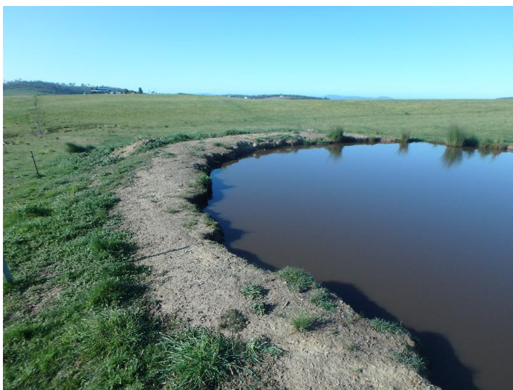
Plate 9: View west at erosion scalds around a farm dam within the study area
