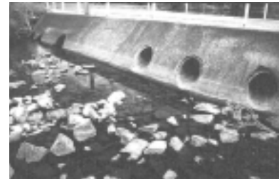
Multi level culverts may allow fish to pass through causeways during low flows
