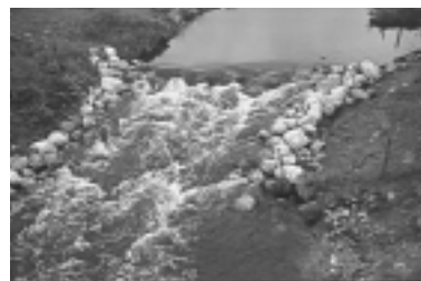
Seek expert advice if installing bed control structures such as rock chutes
