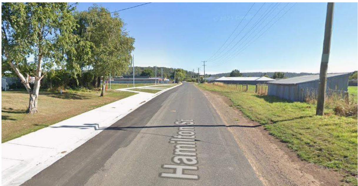
Figure 2-4: Hamilton Street Facing North
