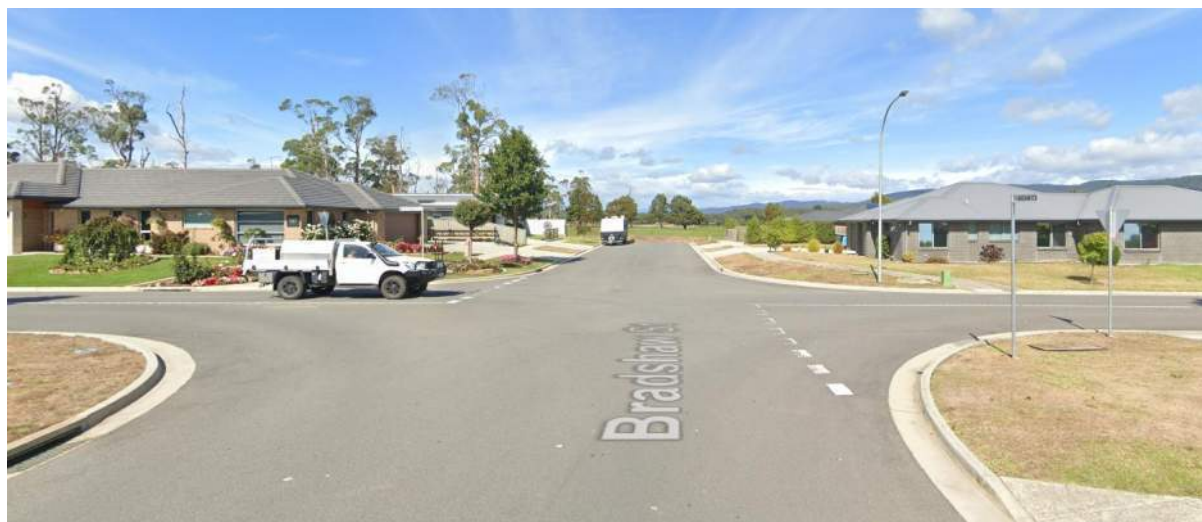
Figure 16: Bradshaw Street at the intersection of Calthorpe Street, looking south towards the subject site
