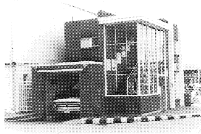
Franklin Wharf : A small-scale building in the Main Space
