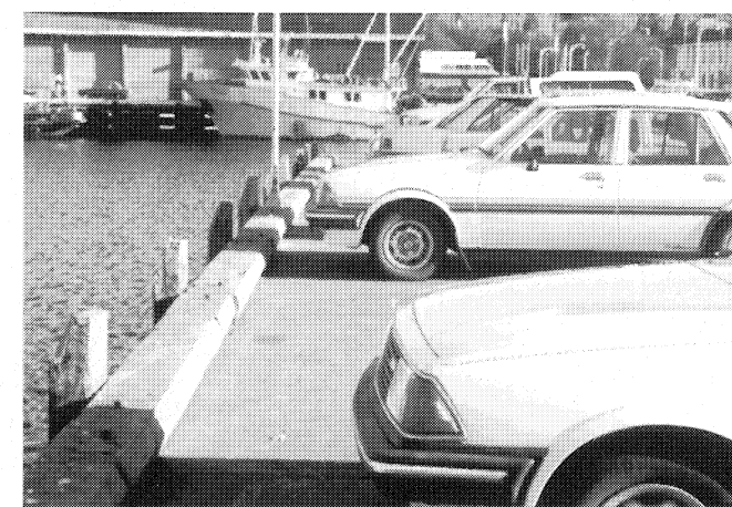
Franklin Wharf: carparking at wateredge interrupting pedestrian movement
