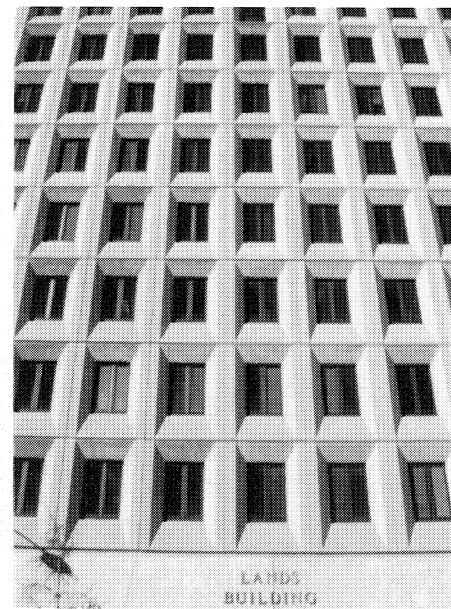
High and Bulky: Lands Building, Macquarie Street
