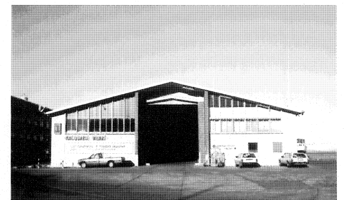
Wharf Shed, Macquarie Wharf No. 1: a free standing building with a slightly ambiguous orientation
