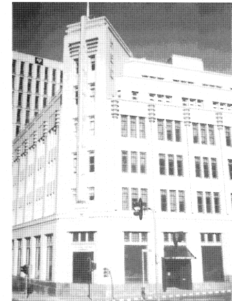
Cnr Davey Street and Elizabeth Street : HEC Building: within an area of government administration
