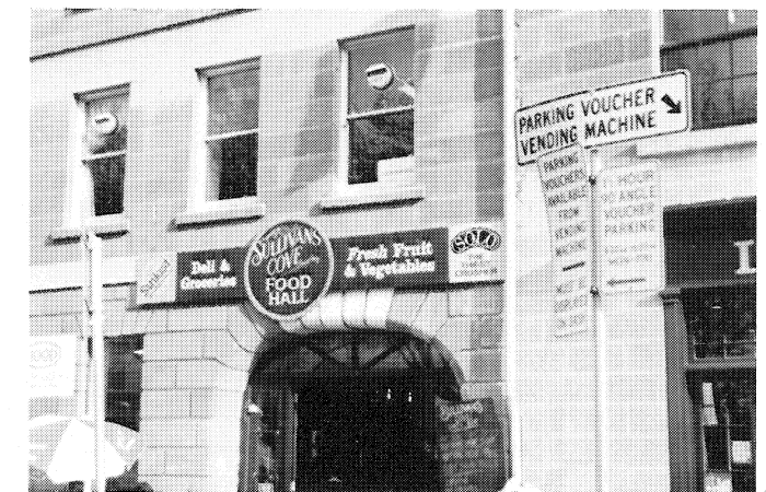
Salamanca Place : too many signs
