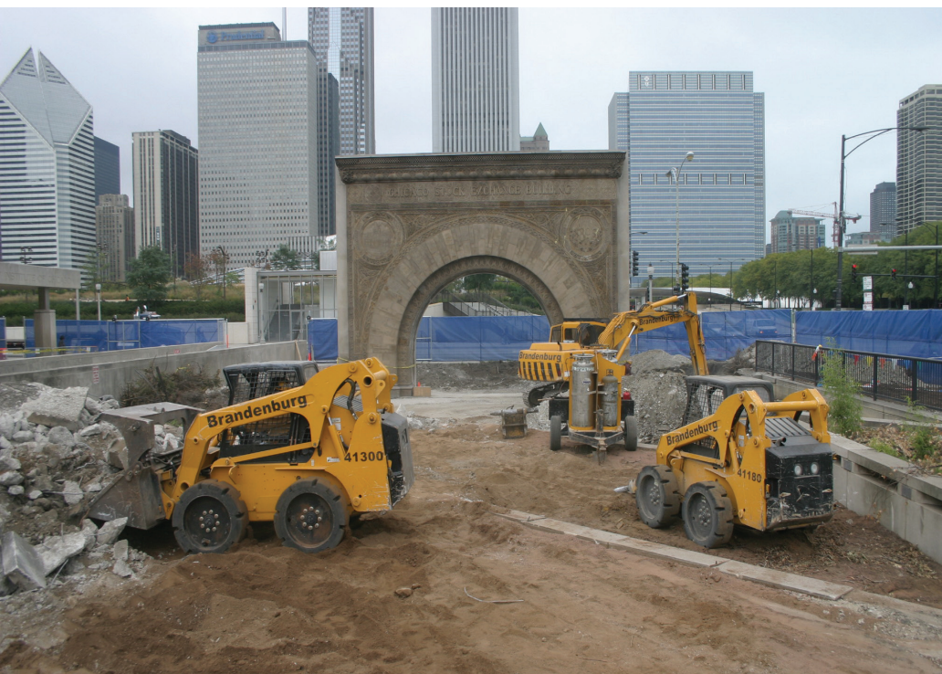
Fig. 8. Site-grading activities near Sullivan Arch next to the Modern Wing addition at the Art Institute of Chicago, 2005.
