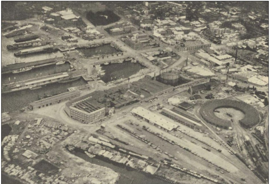
Figure 8: Figure 5.5.5 from Appendix M ( Historical Archaeological Assessment op cit. p48 ) showing a fragmented and inconsistent built edge to Evans Street and inconsistent building form in 1924.
