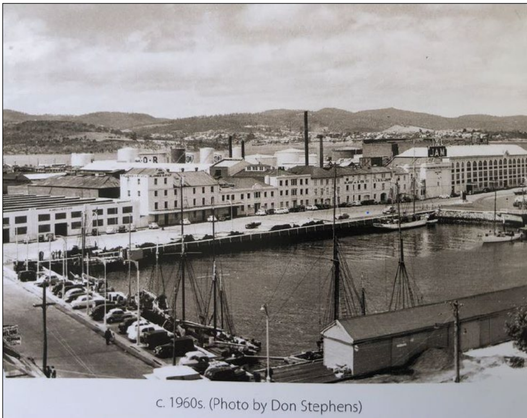
Figure 15: Figure 56 from the 2024 SDP showing a different angle of the additional layer of buildings and roof structures behind the Hunter Street buildings including port - related structures (view from TMAG building). The building on the far left is situated on the former site of a gasometer.
