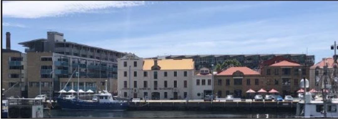
Figure 14: Figure 30 from the 2024 SDP showing a closer view of the additional layer of buildings and roof structures behind the Hunter Street buildings (view from southern side of Victoria Dock)
