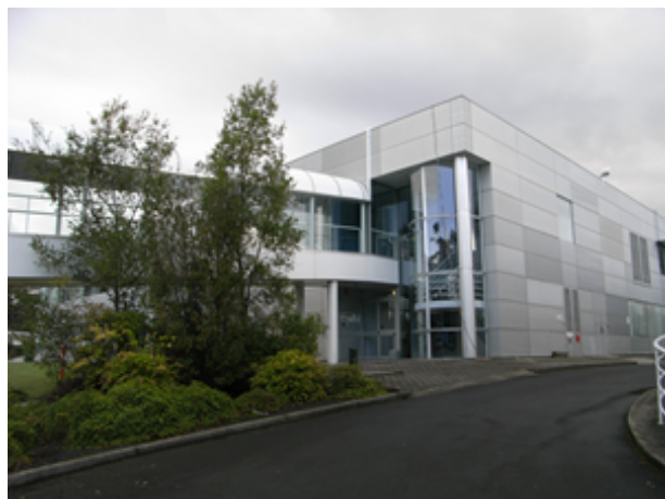
Hurley Building No copyright on file
