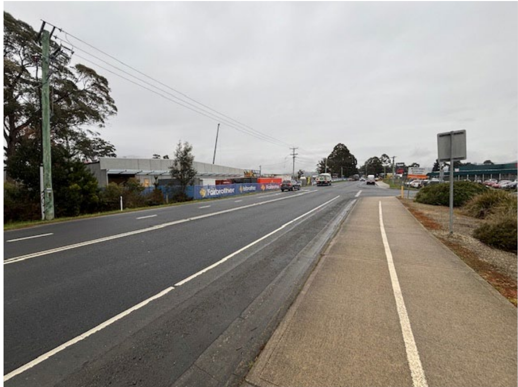
Figure 7 - View looking north along the Channel Highway near the entrance to the AAD campus at [REDACTED]. The new commercial development at 202 Channel Highway is under construction on the left of picture.
