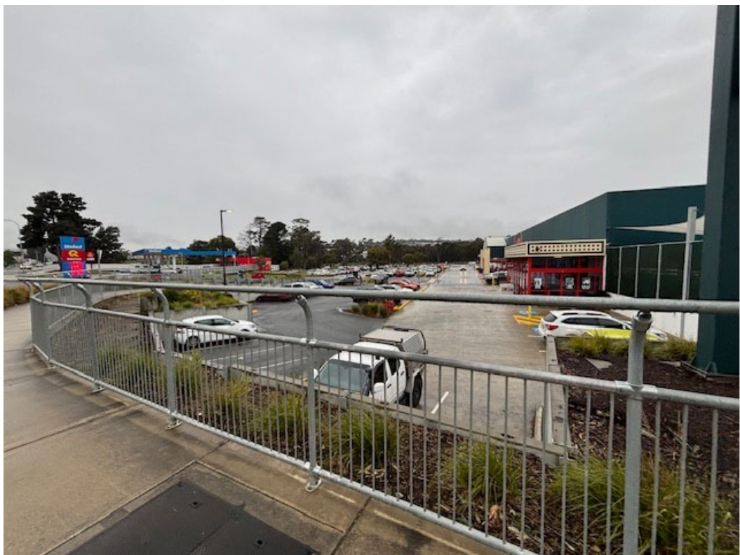
Figure 10 - View looking east from the Channel Highway frontage over the Bunnings site at [REDACTED]. [REDACTED] owned by AAD Nominees is located behind the carpark in the center of the picture.
