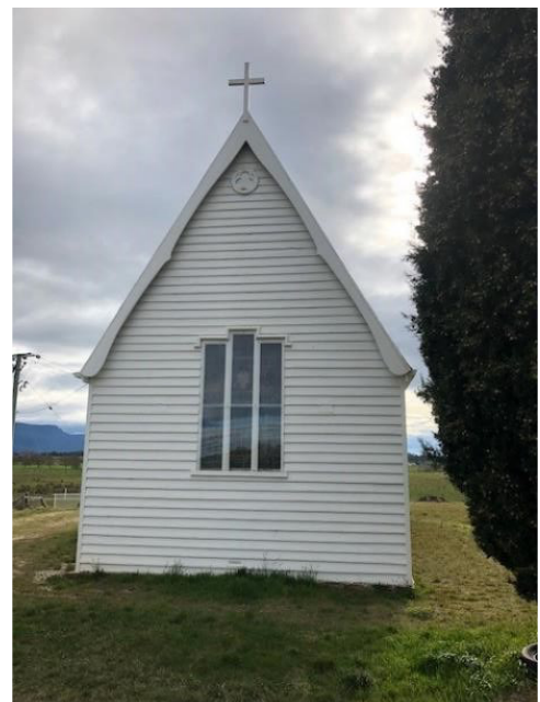
East side of the building showing the steep gable roof with modestly shaped barge boards and narrow window frames. The narrow windows forms have been coupled together to form a wider window.
