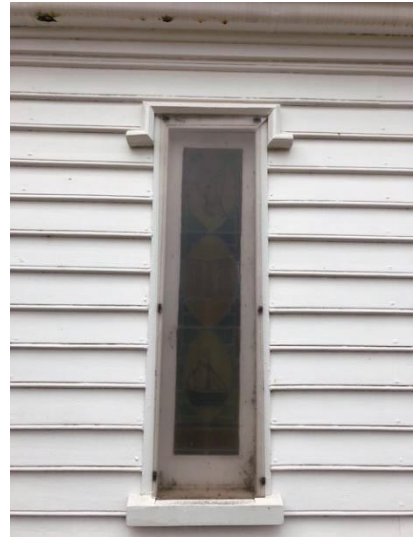
View of narrow side window with bottom beaded timber weatherboards
