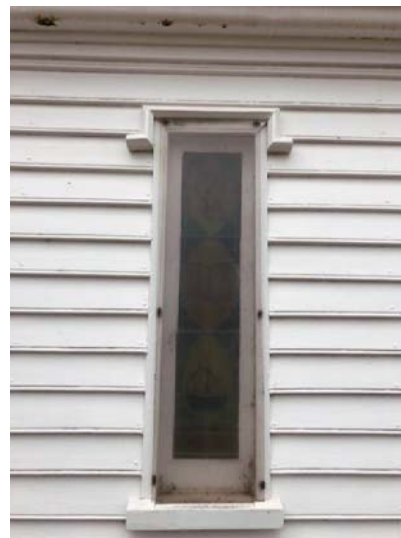
View of narrow side window with bottom beaded timber weatherboards
