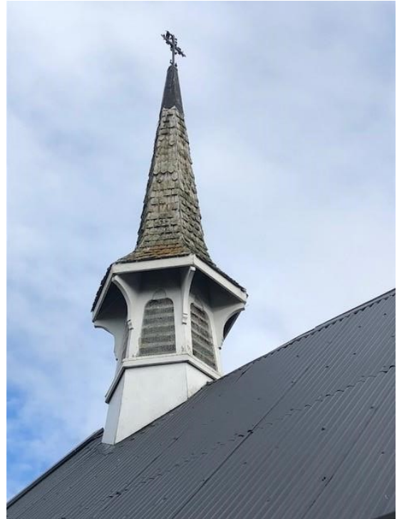
Hexangular Belfry with timber louvre bell screen, Huon pine shingle roof and decorative iron finial
