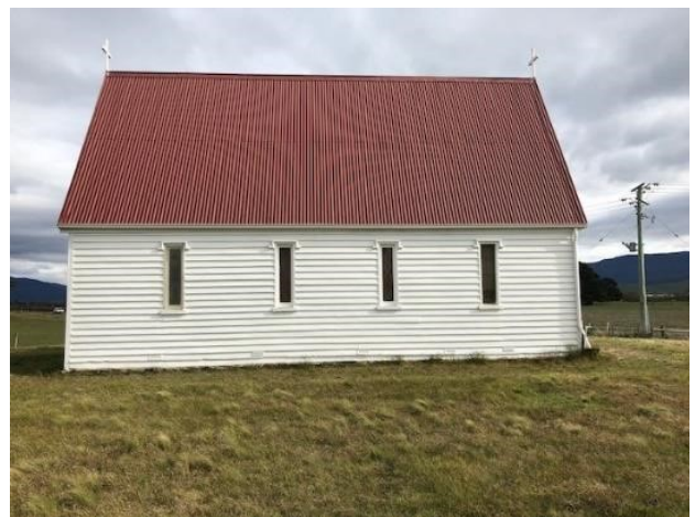
North side of the building with 4 equally spaced narrow windows. The weatherboards extend to the ground with no visible foundation wall
