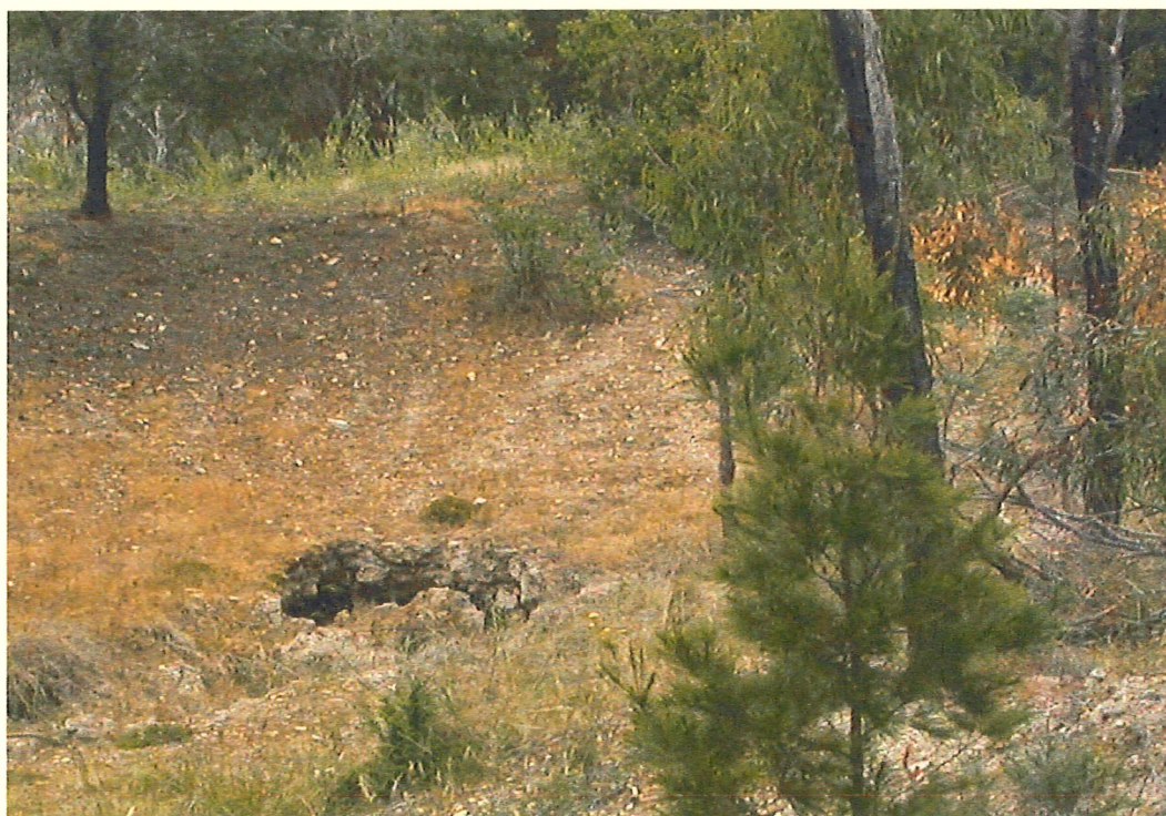
Plate 3 Tunnel erosion in upstream face of dam on proposed lot 2
