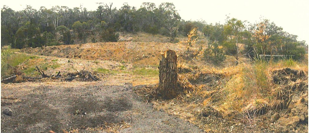
Plate 5 Fill embankment on proposed lot 2 (background) and slope grooming on proposed lot 1
