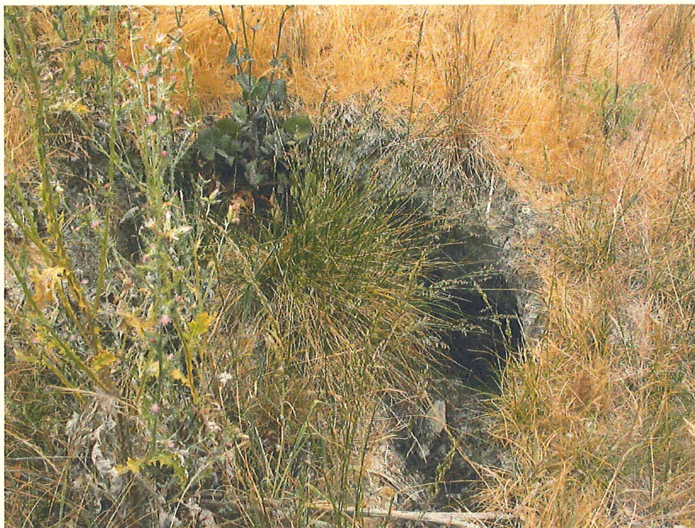
Plate 4 Tunnel erosion in upstream face of dam on proposed lot1.
