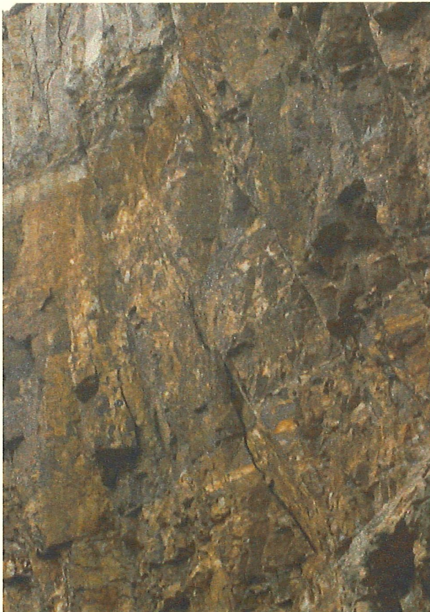
Plate 11 Separation along a defect has resulted in a column of rock that is almost certain to topple into the floor of the quarry.
