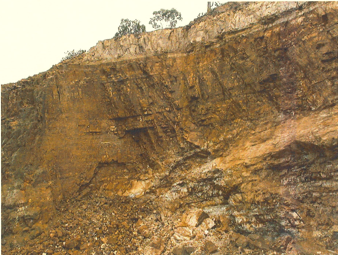
Plate 9 Defects dipping out into the quarry allow present a hazard of planar rock failures
