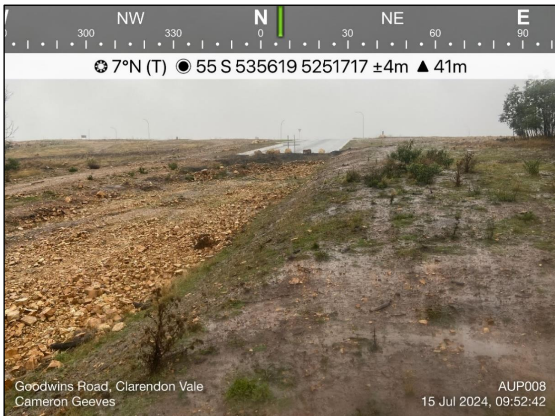
Plate 2. Looking north from the lot boundary towards newly created road on the adjacent subdivision. This road is proposed to continue through the lot to link with Goodwins Road.
