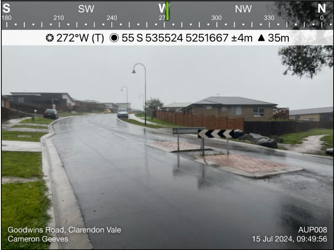
Plate 7. Looking back up Goodwins Road. Low threat vegetation.
