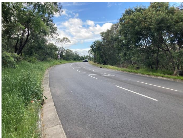
Figure 26: Goodwins Road, east approach to Access #1
