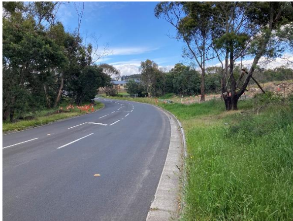
Figure 4: Goodwins Road (facing west)
