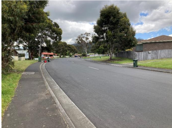
Figure 8: Mockridge Road (facing north)
