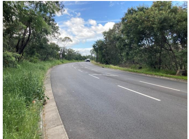
Figure 5: Goodwins Road (facing east)
