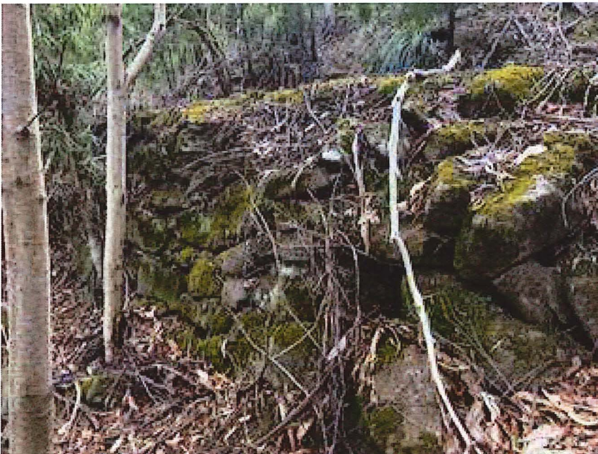
Evidence of old hand laid roadworks along the forest reserve road at the end of [REDACTED] [REDACTED] used to extract timber(pre-1900's)
