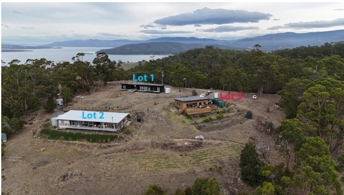
Figure 1 – Aerial view of subject site showing existing development (Lots 1, 2 and 3)
