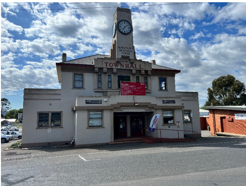
Photograph 1: View of the front of the Campbell Town Hall from High Street
