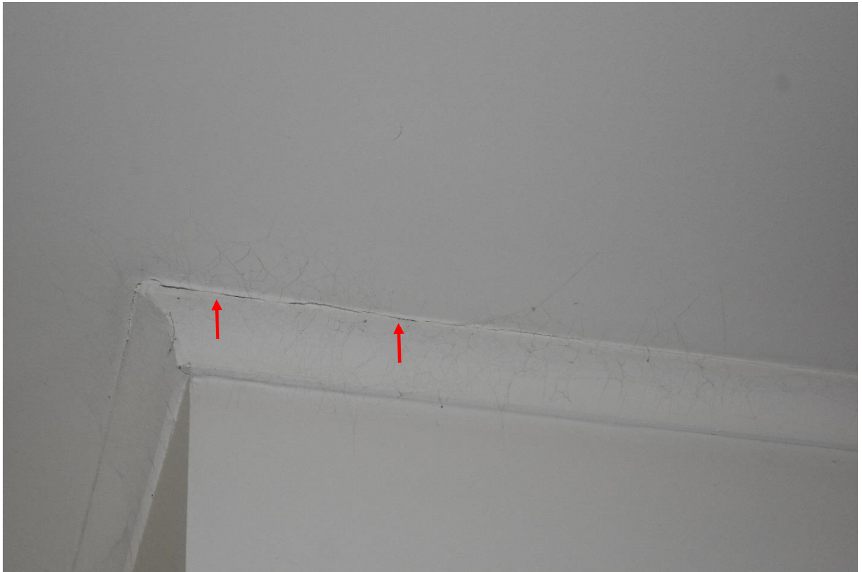
CRACKING IN LIVING ROOM CEILING
