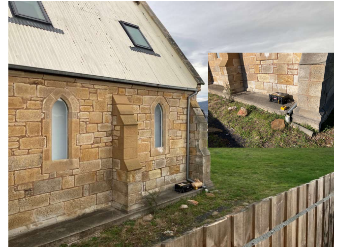
Figure 1. Vibration monitoring at THR 624 St Mary's Church, 18-20 Old Main Road, Bridgwater
