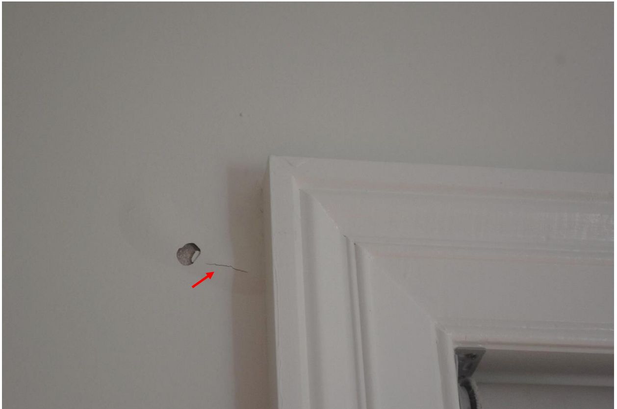
CRACKING IN OFFICE WALL
