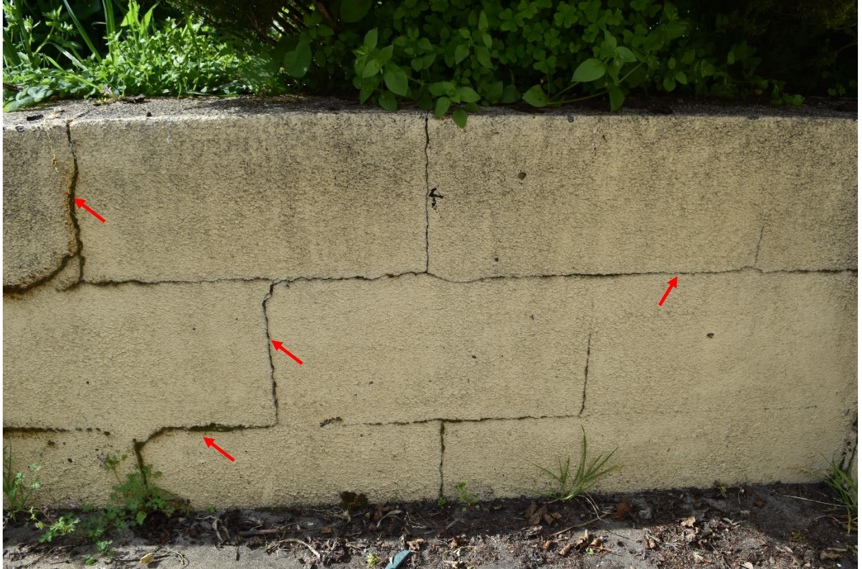
CRACKING IN RETAINING WALL- 1mm GAP APPROXIMATES
