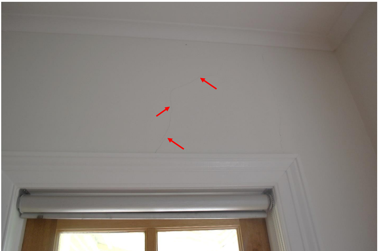
CRACKING IN OFFICE WALL
