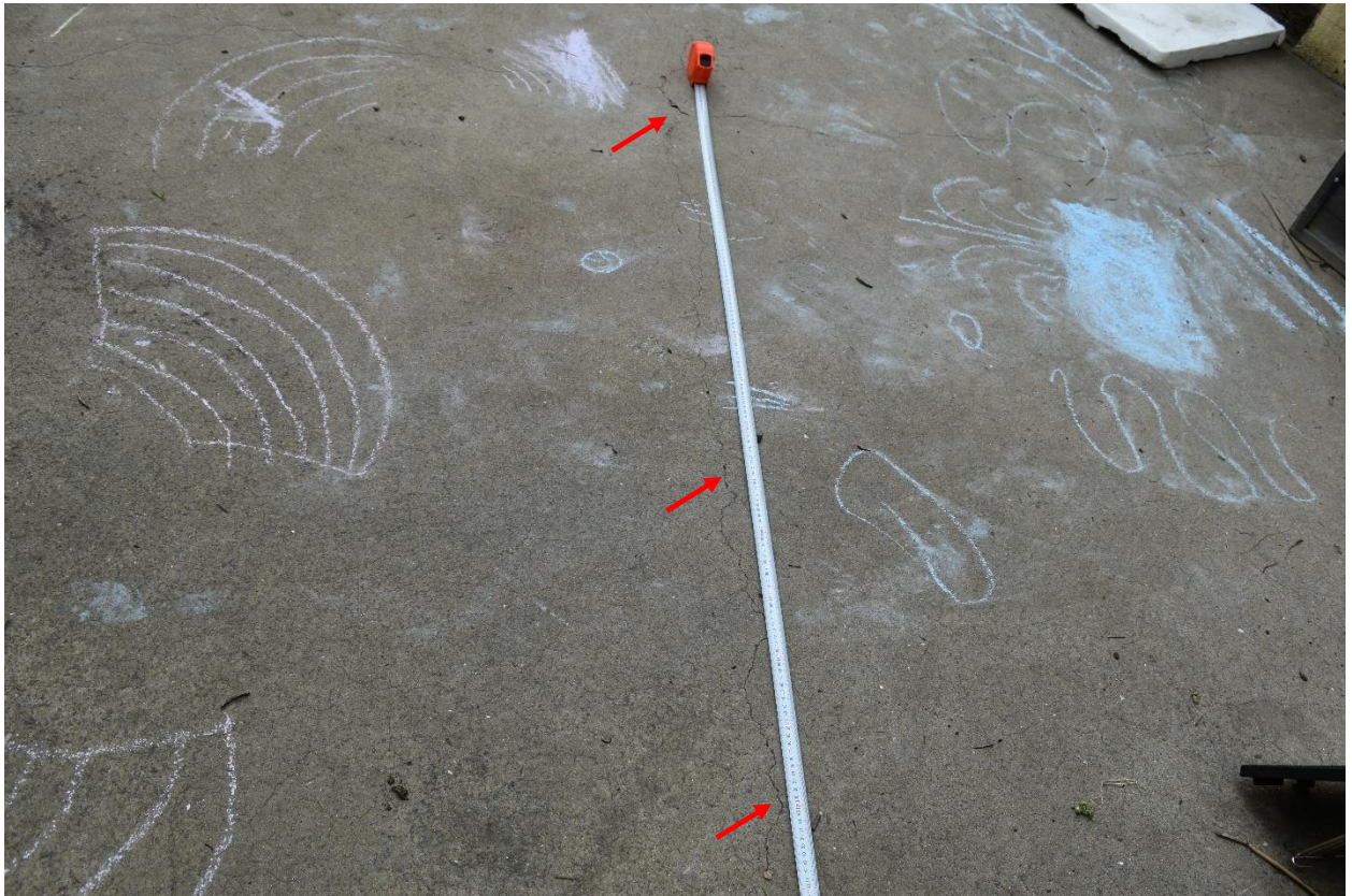
CRACKING IN CONCRETE SLAB REAR OF BUILDING- 2.64m IN LENGTH WITH GAP OF 1mm APPROXIMATES
