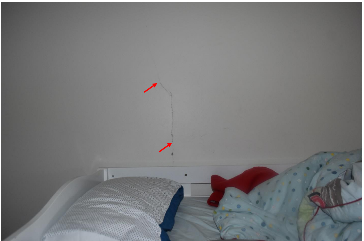
CRACKING IN BEDROOM WALL
