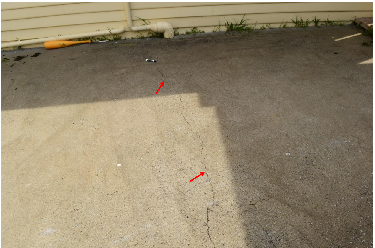
CRACKING IN CONCRETE SLAB REAR OF BUILDING- 4m IN LENGTH WITH GAP OF 1mm APPROXIMATES
