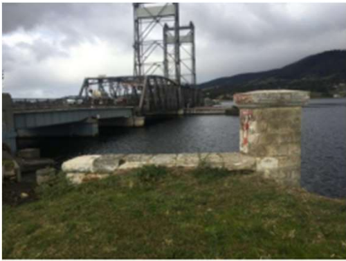
Figure 9: Western side of causeway, below the rail line, showing the sand and mudstone retaining wall, looking south.
