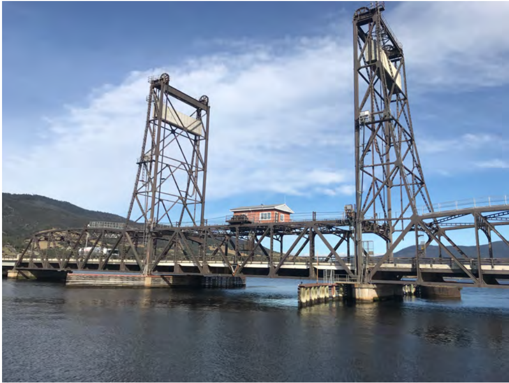
Photo 5 The lift span required for vessels passing under the existing Bridgewater Bridge.
