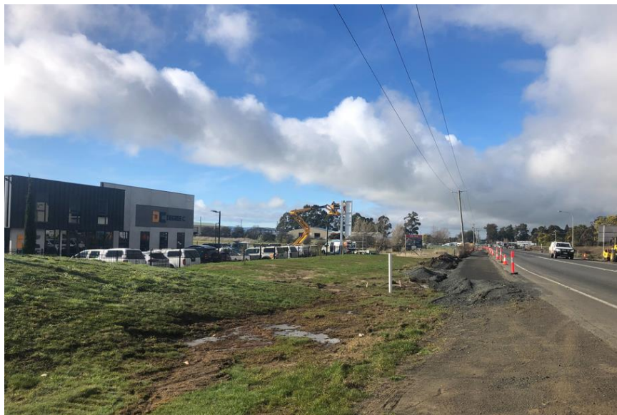
Figure 2 - New commercial building located at 6 Richard Street, 150m from site. Photo take from Evandale Road.
