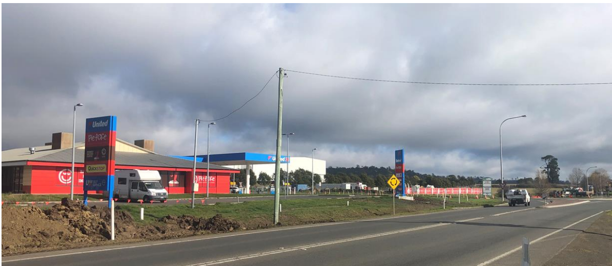
Figure 4 - United Petroleum Service Station, located on corner of Evandale Road and Translink Ave
