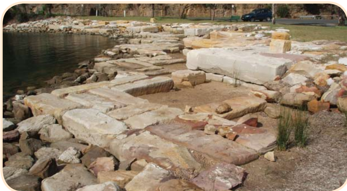
Figure 15.5 Best practice rock revetment that is aesthetically pleasing and provides intertidal habitat at Bobbin Head, Cowan Creek, Hawkesbury River, NSW. © Daniel Wiecek, DECCW
