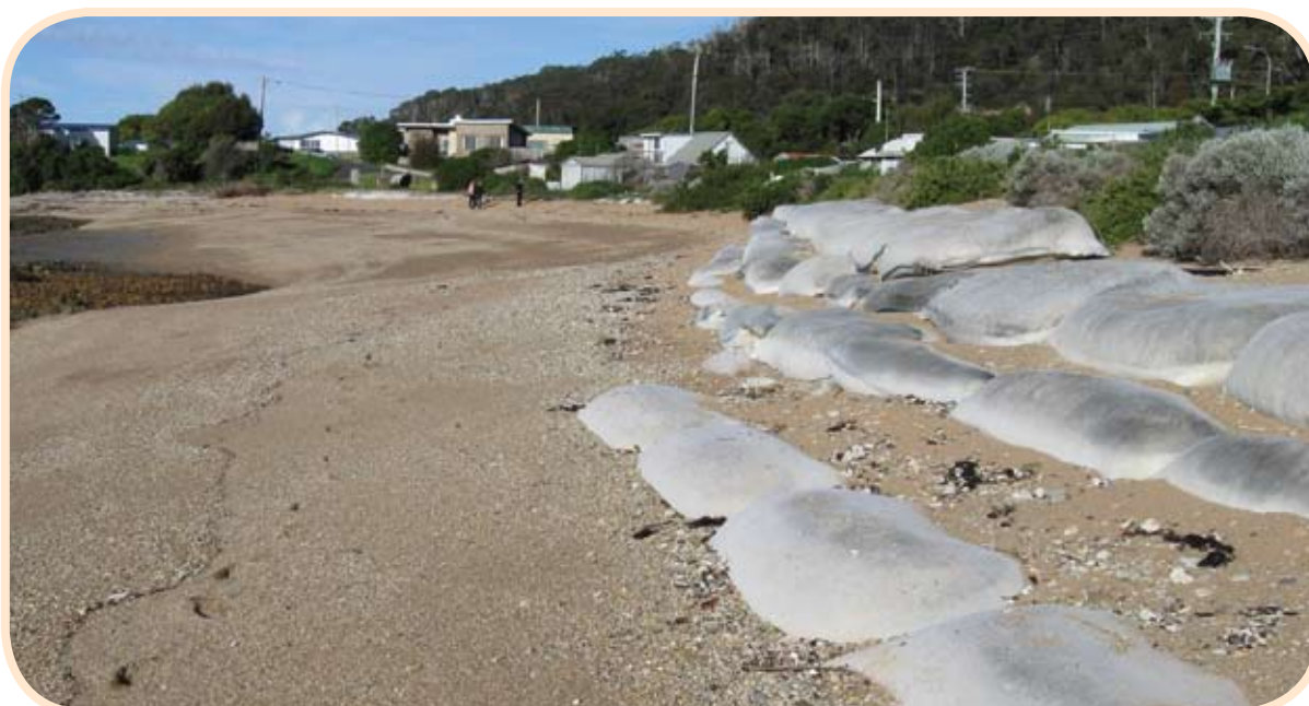
Figure 15.10 Geotextile sand container revetment at Blythe Heads in north-west Tasmania. © Jocelyn Phillips
