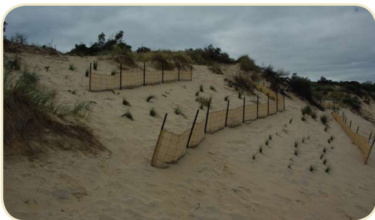
Figure 6.5 Geotextile dune-forming fence erected near surf club in South Australia is helping to trap sand and discourage access whilst plantings of dune grasses become established. © Leah Page
