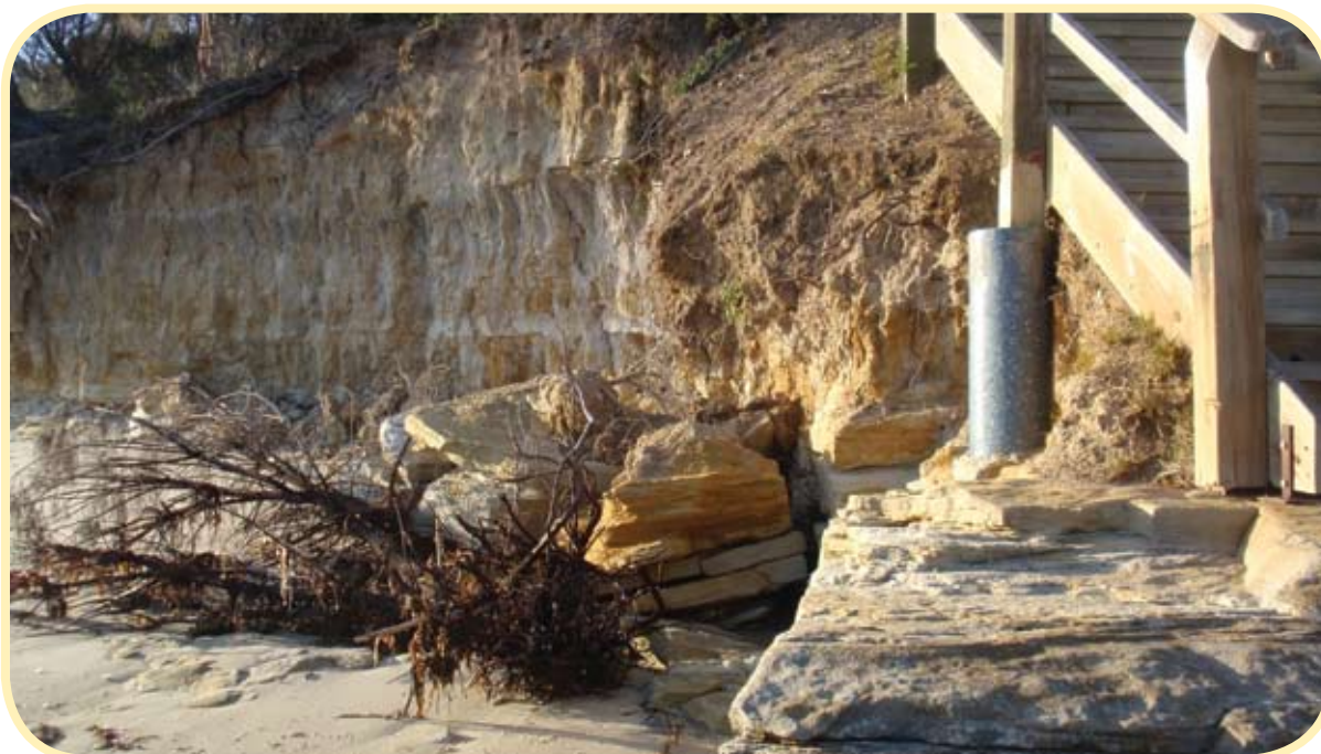
Figure 13.10 Steps encroached on by erosion were becoming unsafe and have since been removed. © Chris Sharples
