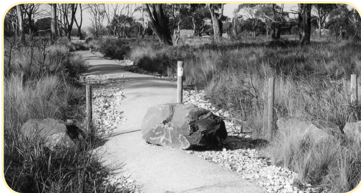
Figure 13.17 Large rocks and bollards can be used to stop vehicle access onto a walking track. Source: Community Coastcare handbook (Thorp 2005)
