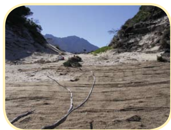
Figure 13.7 Laying geotextile protects Aboriginal heritage material by minimising future disturbance to the midden. © Aboriginal Heritage Tasmania
