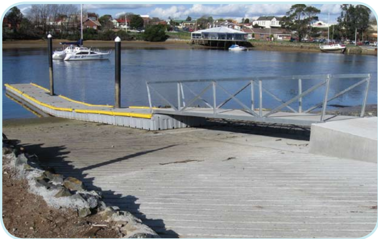
Figure 14.2 The boat ramp at Ulverstone has a floating pontoon to minimise impacts on the sea floor and interference with sand transport along the shoreline. © Jocelyn Phillips
