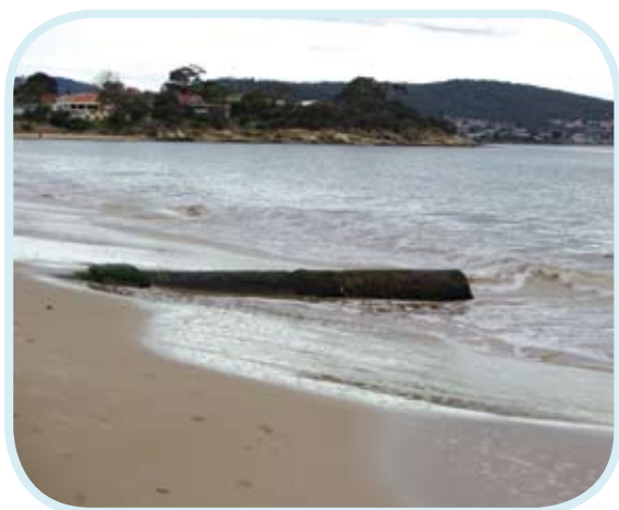
Figure 12.2 Inappropriately sited pipeline on beach is hazardous and looks unsightly. © Leah Page
