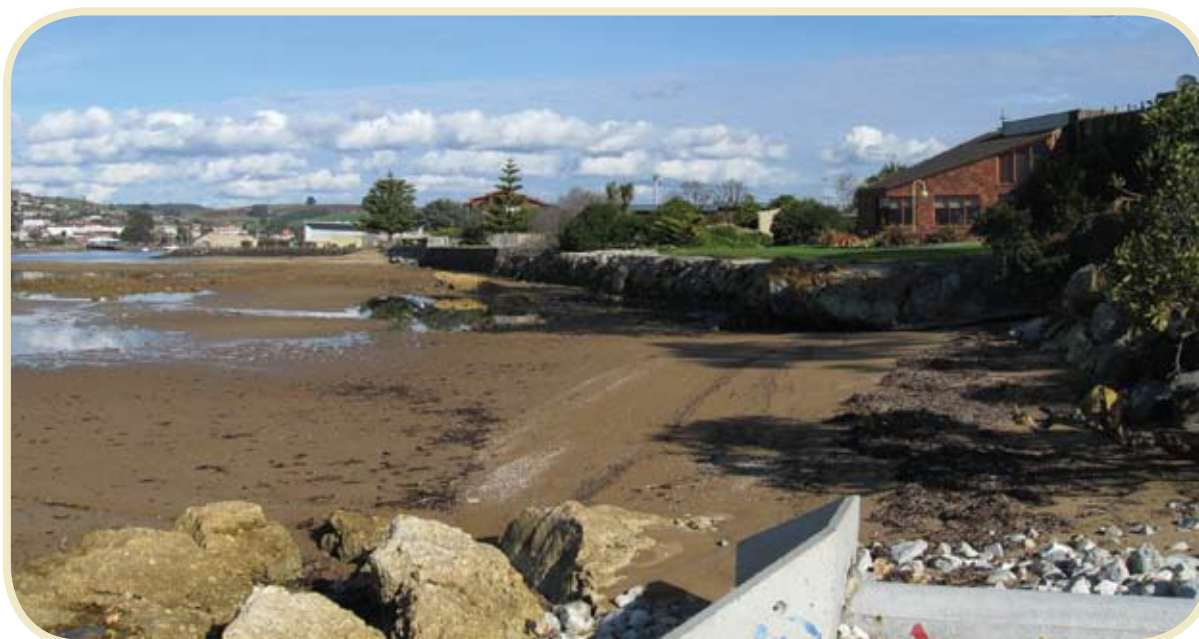
Figure 6.8 The river training walls at Ulverstone are not preventing the build up of sediment as intended. © Jocelyn Phillips
