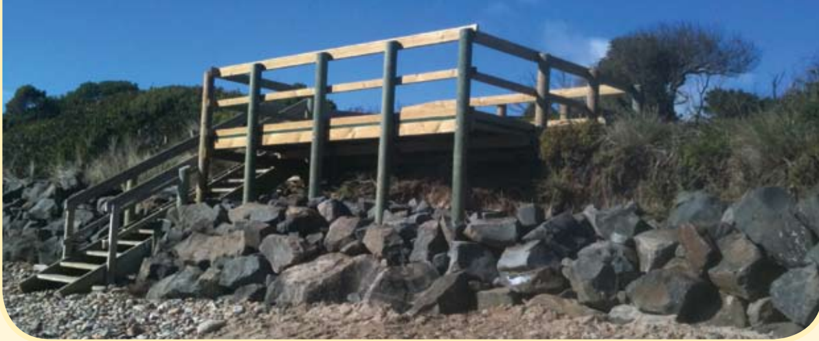
Figure 13.15 The viewing platform at Turners Beach incorporates mesh flooring to allow water, air, sand and light to penetrate to the vegetation below. Its location on the foreshore required the installation of rock to protect the structure from wave action. Geotextile sand containers or local rock material are other options. © Justin Smith
