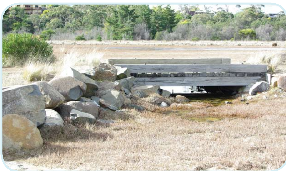
Figure 12.10 Small-scale private crossing over saltmarsh area - whilst in poor condition, it does allow the free passage of water. © Leah Page
