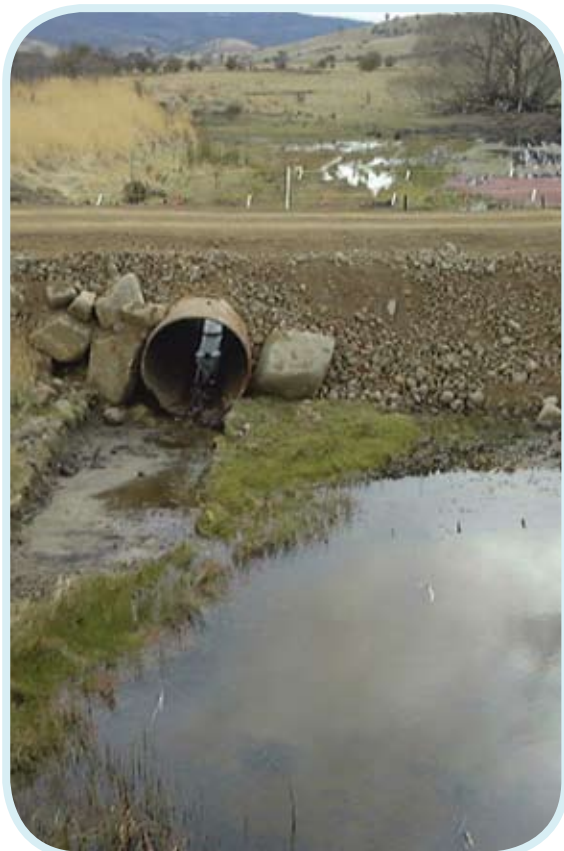
Figure 12.11 Inappropriate culvert is sited poorly and does not allow passage of fish at low flows. Source: Wetlands and waterways manual (Gallagher 2003)
