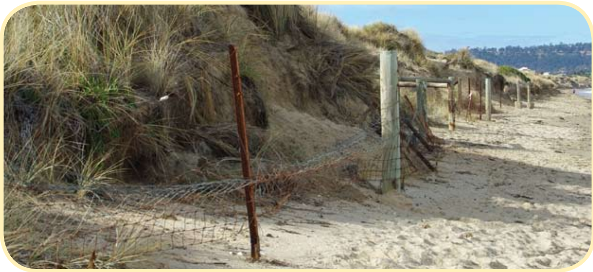
Figure 13.19 This poorly maintained coastal fencing looks unsightly and has become a hazard to the public. A simple, cheaper fencing alternative such as a dripline fence on the seaward side would be more appropriate. © Leah Page
