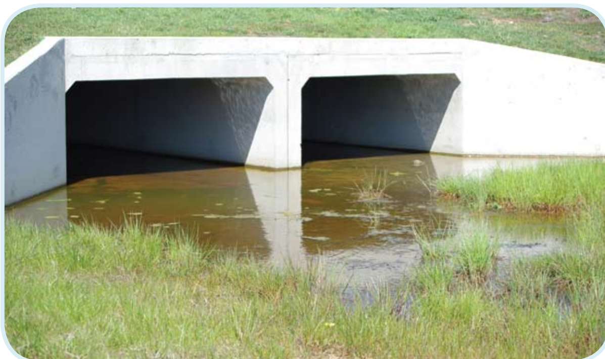
Figure 12.12 Wherever possible box culverts are best as they can accommodate high flows and are open at the bottom to allow for natural sediment beds. © Leah Page
