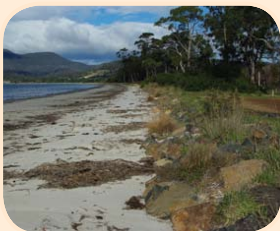
Figure 15.9 The rock revetment at Raspins Beach on the east coast has trapped sand and is stabilised by vegetation. © Leah Page
