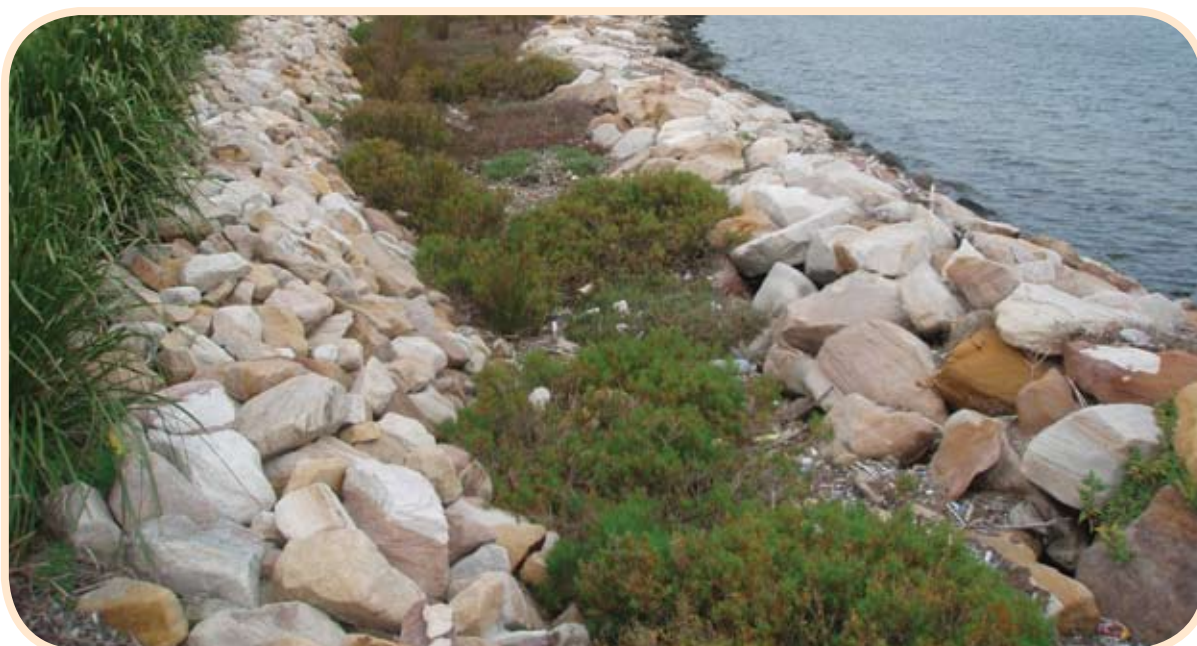
Figure 15.8 Rock revetment with bench in Claydon Reserve, Kogarah Bay, Georges River, NSW. © Daniel Wiecek, DECCW
