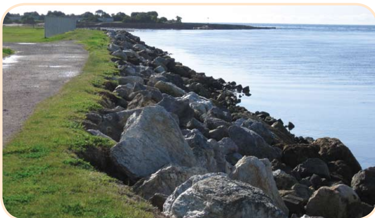
Figure 15.6 Revetment degradation due to either scour by overtopping waves or seepage loss of fill. © Jocelyn Phillips
