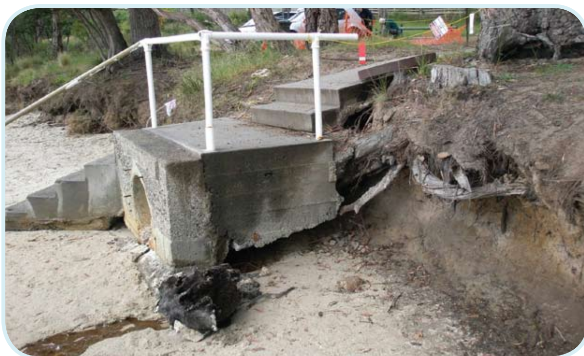
Figure 12.1 Eroded stormwater outlet associated with public access has become a hazard. © Kevin Phillips
