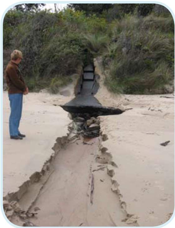
Figure 12.3 Inappropriate siting of stormwater outfall on beach causes scouring and restricts pedestrian access. © DPIPW
