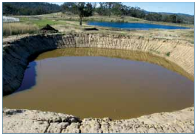
Figure 32. The dam in the foreground has been constructed from dispersive clays. Note the rill erosion and cloudy brown colour of water in foreground, compared to the blue colour of the dam constructed from non-dispersive soils in the background.
