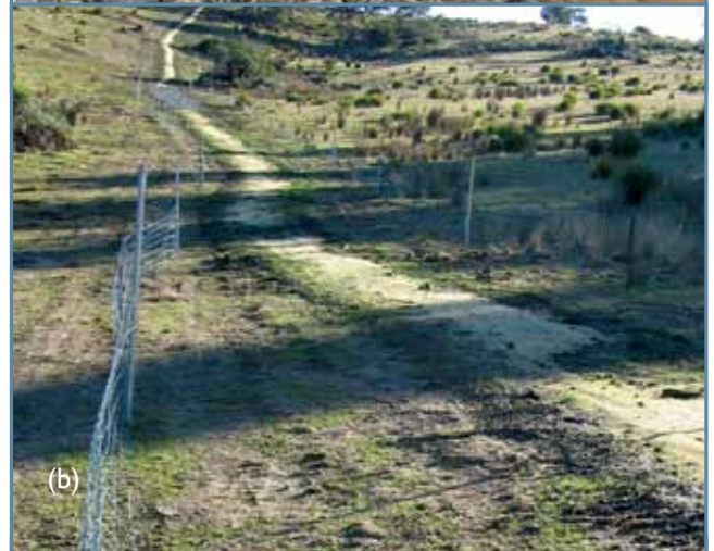
Figure 36. Examples of tunnel erosion control (a) Poor technique. Rock rap is usually an inappropriate erosion control technique for dispersive soils. Normally rock barriers work well to trap sediment and reduce erosion. However in dispersive soils, hard surfaces such as rock are quickly bypassed i.e. upper corner of the rock structure (b) Excellent technique. Note the entire repaired area is fenced, and the whole length of the repaired tunnel is covered with topsoil and jute cloth. Sand barriers have been constructed every 20 meters down the slope.
