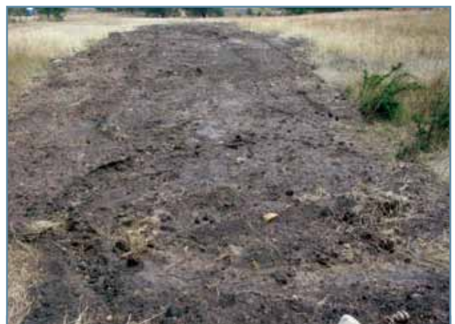
Figure 37. Good technique. Topsoil mounding, reclaimed tunnel erosion, Brighton. Note the width of earthworks required to fix a 50cm wide tunnel, and the raised profile to shed surface water. Jute cloth would prevent surface erosion until vegetation has established.
