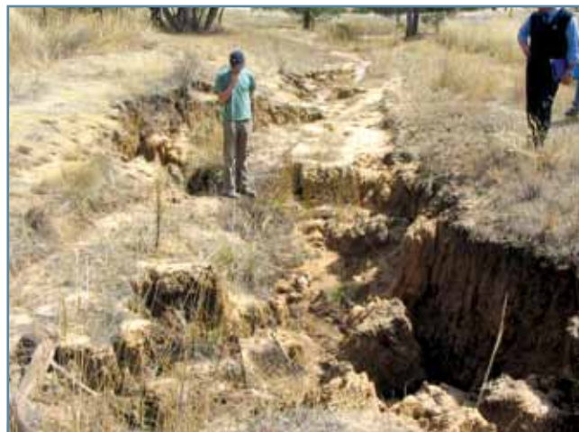
Figure 24. Tunnel erosion resulting from construction of a stormwater culvert in dispersive clay derived from Triassic sandstone, Brighton.
