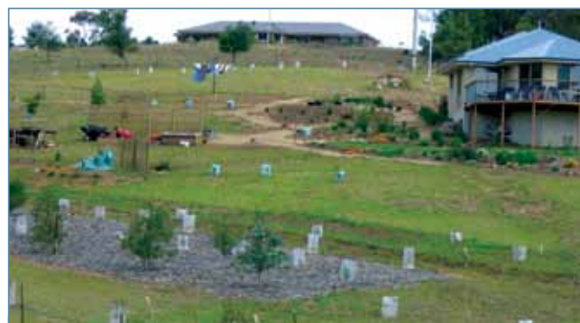
Figure 30. Ozzi Kleen single tank (Aerated Wastewater Treatment System) for treatment and disposal of sewage and grey water. Raised – mulched area in foreground is being used for effluent disposal from the house in background.
