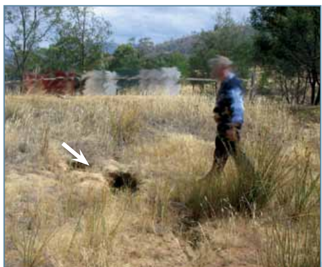
Figure 33. Typical small dam failure. Note piping through the side wall of the dam. This dam was constructed using dispersive clays derived from Triassic sandstone.
