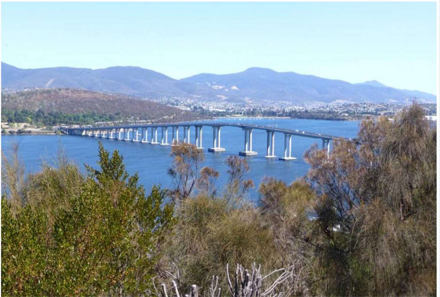
Figure 21 TASMAN BRIDGE Source: https://www.ourtasmania.com.au/tas-history-bridges.html accessed June 2025
