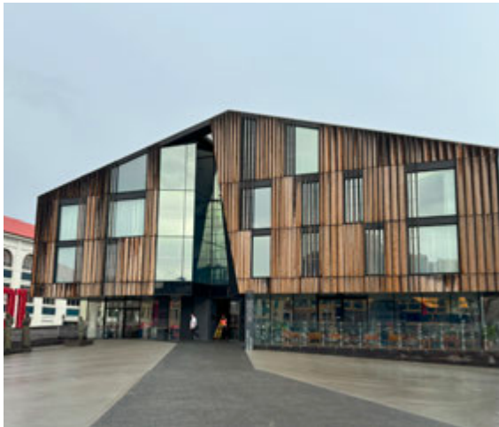
Figure 137: The timber facade of MACq 01 Hotel
