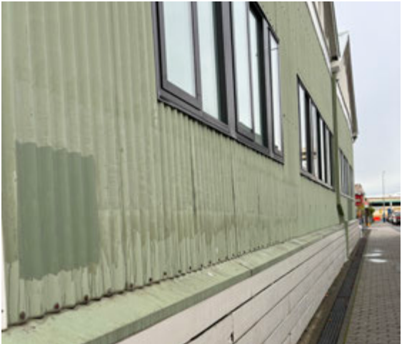
Figure 138: The corrugated iron Goods Shed ‘
