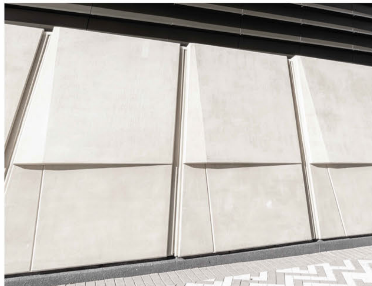
FT06 PRECAST CONCRETE WITH VARYING PANEL TYPES
