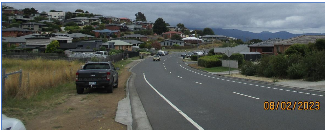
Photograph 5.1 – Typical Cambridge Road standard
