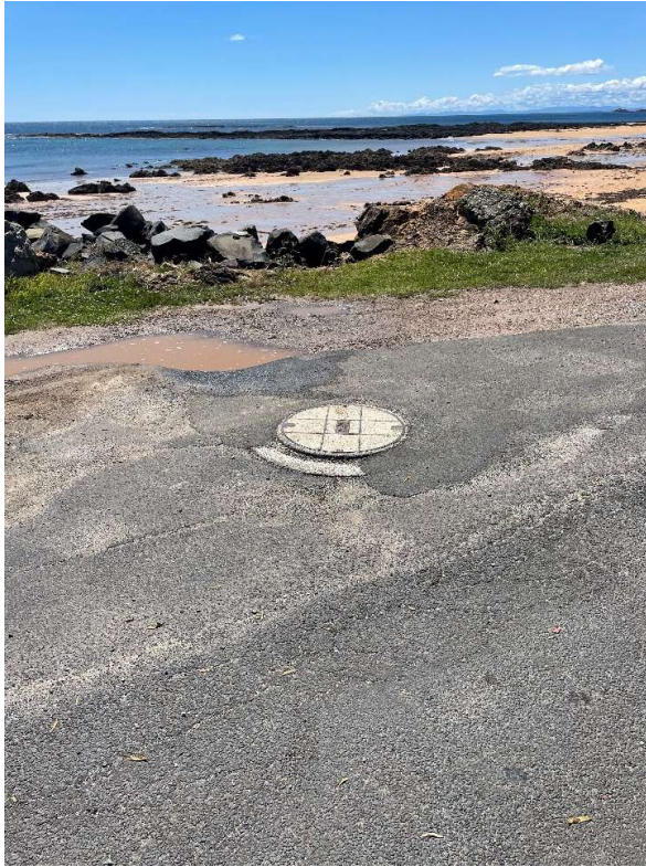
Image 6: Manhole ~50m upstream from SPS (emergency overflow point)
