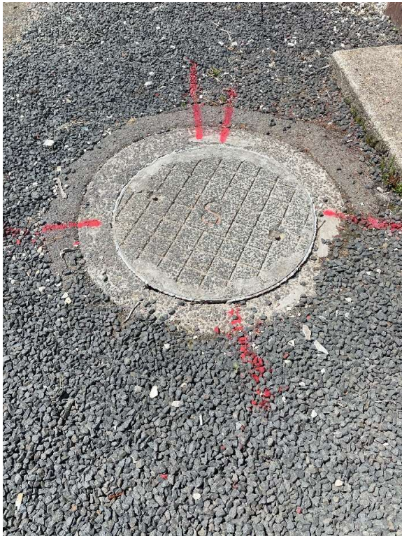
Image 5: 3 of 3 Manholes on inlet side of SPS
