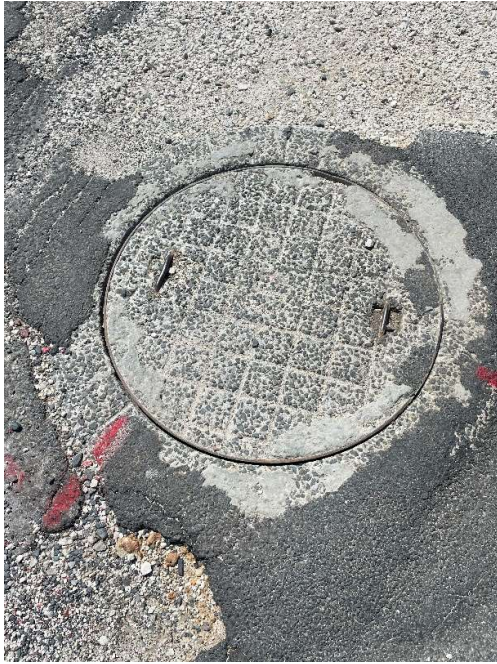
Image 3: 1 of 3 Manholes on inlet side of SPS
