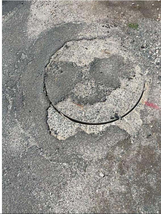
Image 4: 2 of 3 Manholes on inlet side of SPS
