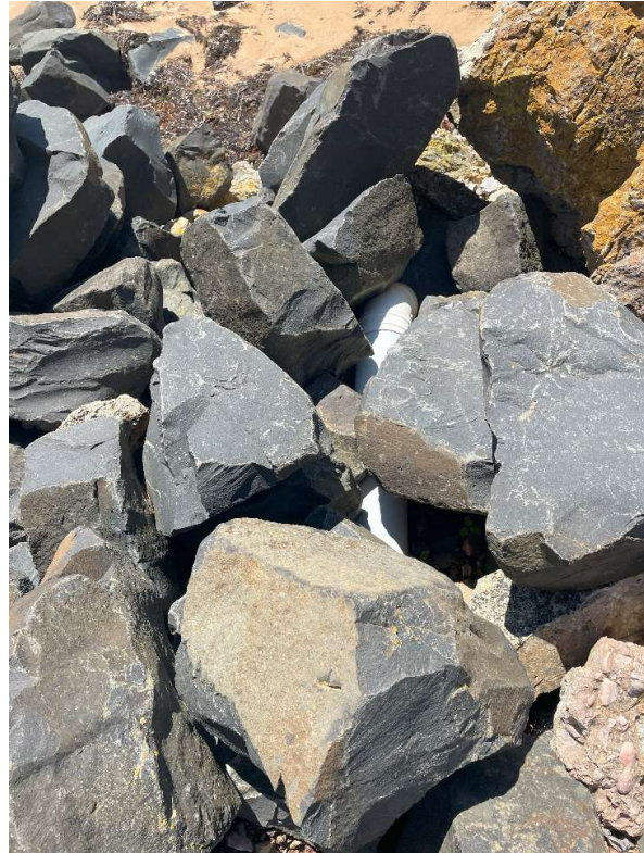
Image 7: White PVC pipe overflow point to Johnsons Beach
