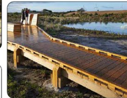
Bridge with kick rail
