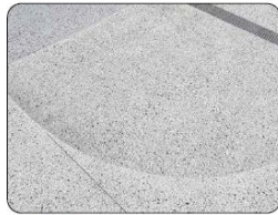
Formal paths Exposed aggregate concrete defines the more formal routes. At 4m wide, these are designed to accommodate both cyclists and pedestrians, linking into the broader shared path network.
