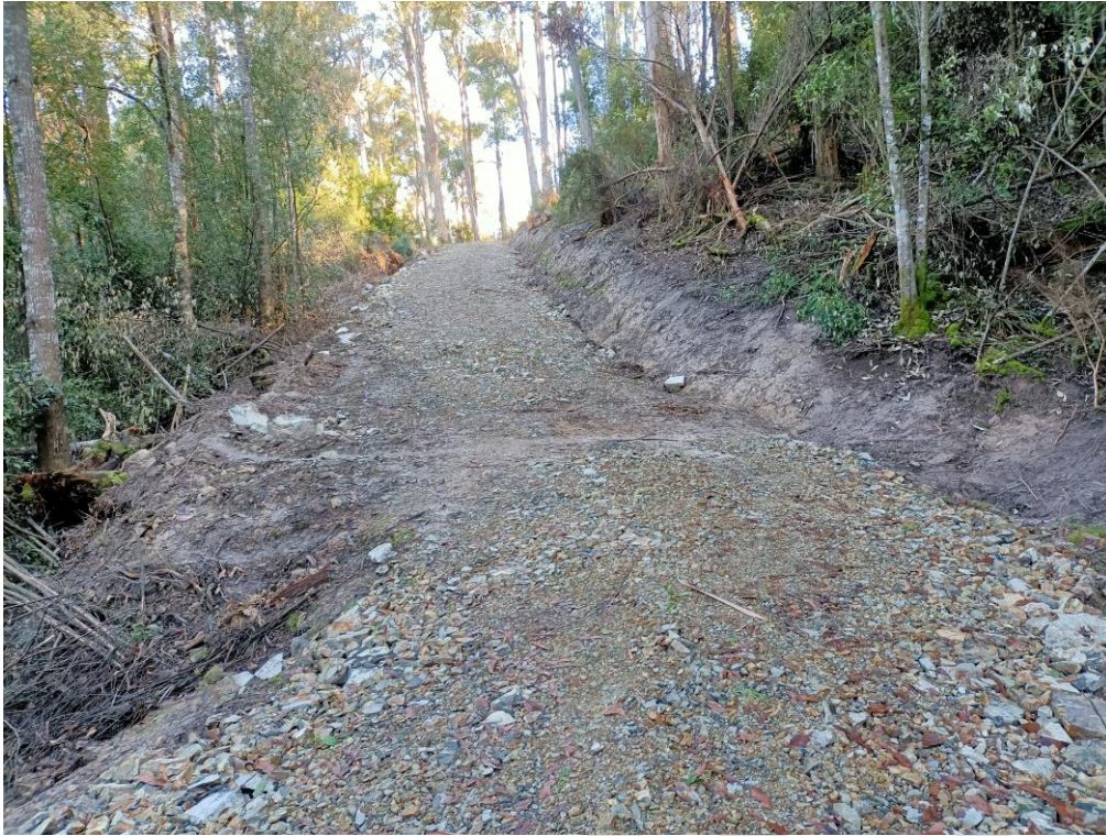
Figure 12 - Image of upgraded internal access within the allotment located within WOB veg community (CH250).
