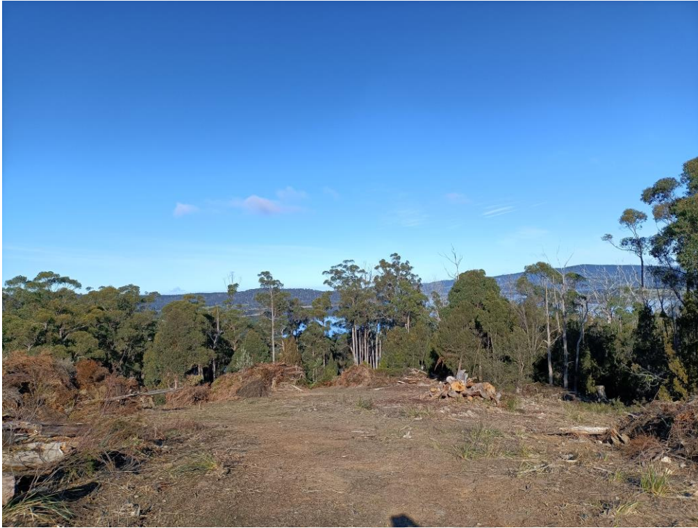
Figure 16 - Image showing extent of clearance and conversion in the central section of the previously cleared area located in the north-west corner of the allotment.
