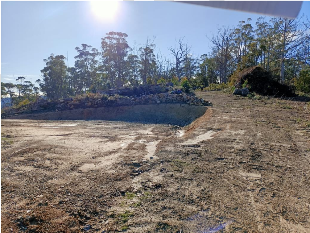
Figure 17 – Image showing extent of existing works and clearance and conversion of vegetation in the northern section of the previously cleared proposed development site.
