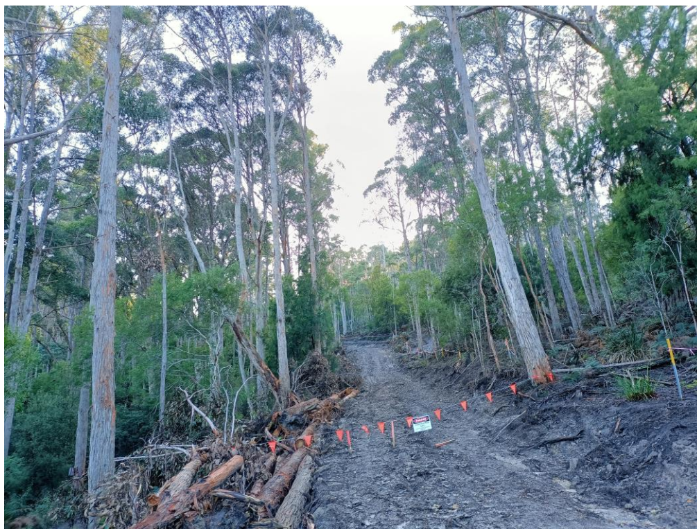
Figure 8 – Image showing the new section of access within the Reserve Road corridor (CH700) within DOB transitioning to WOB.
