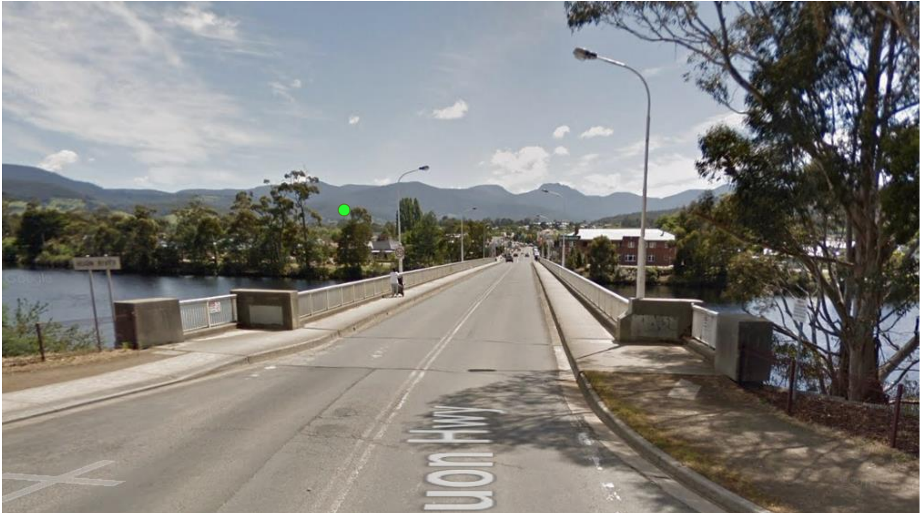
33. Huon river bridge –visible at distance is 8.6km and non-prominent.
