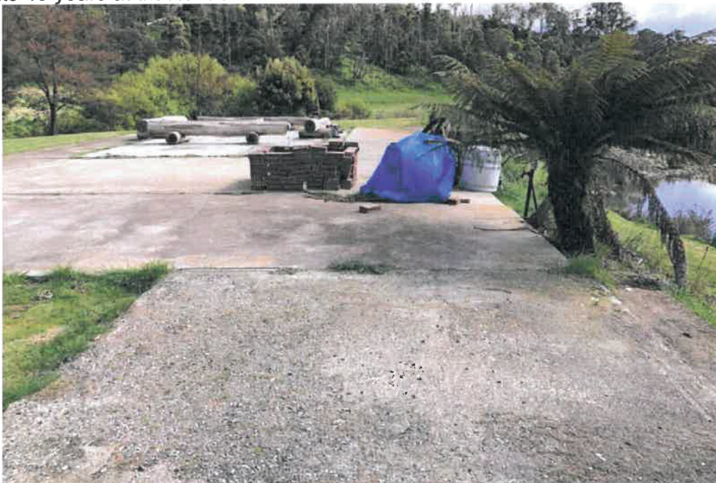
Shack slab level at RL 5.3
