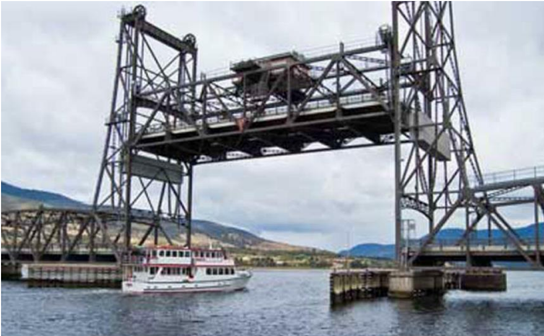
Figure 4 – Existing Bridge with lift span elevated (photo by Ian D Cooper)
