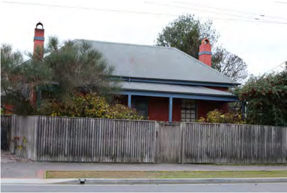
Residential dwelling within retail zone (Main Road)
