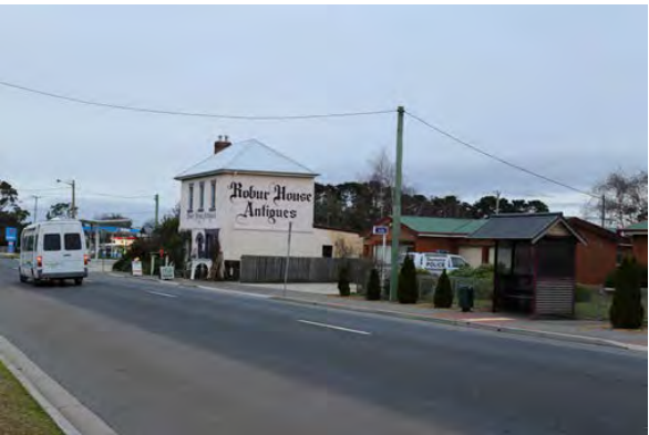
View looking south along Main Road
