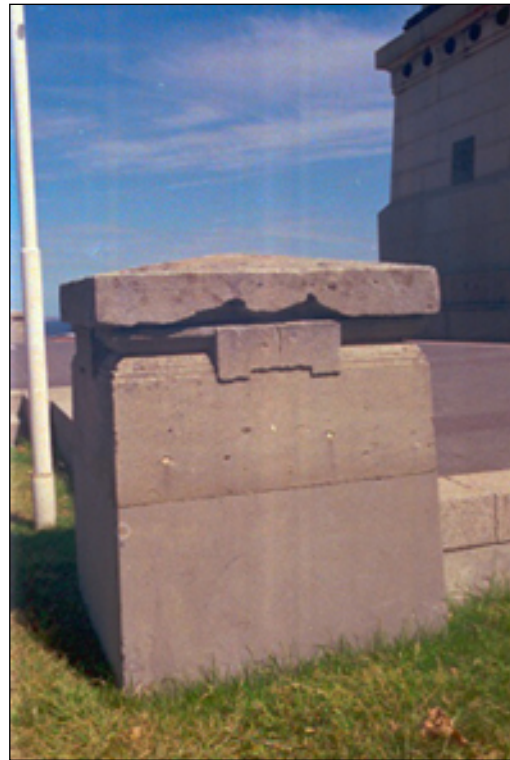
Figures. 25 & 26 . Terrace corner post and paving with variable colours and damaged northern corner post.
