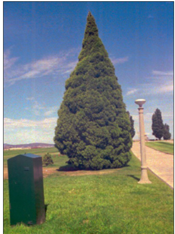
Figure 43. Power box at north western end of Cenotaph Avenue.
