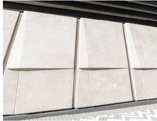
FT06 PRECAST CONCRETE WITH VARYING PANEL TYPES
