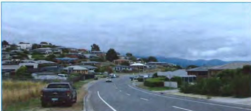
Photograph 6.3A – Available sight distance to the left (150 metres)
