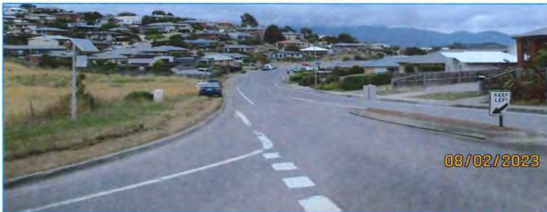
Photograph 5.4A – Available sight distance to the left
