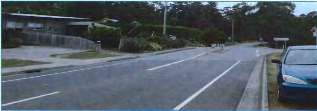
Photograph 6.3B – Available sight distance to the right (150 metres)
