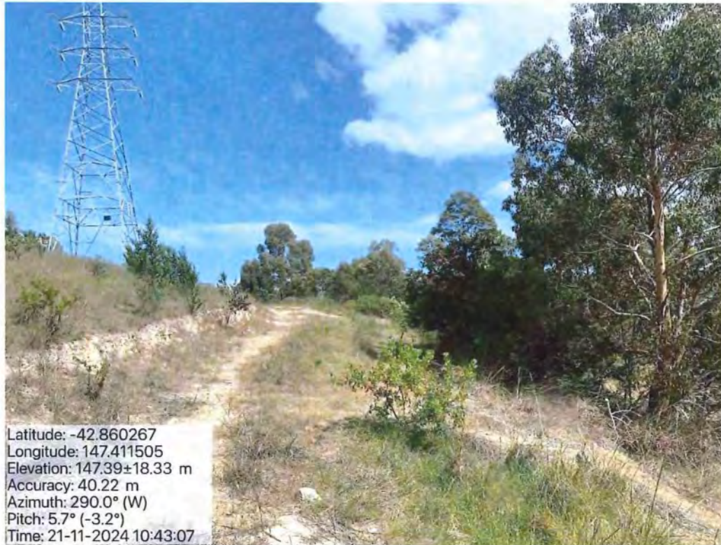
Photo 13 - Fire Trail and HV Lines on the south west boundary of the site (Clarence Waste Transfer Facility to the left) viewing north.
