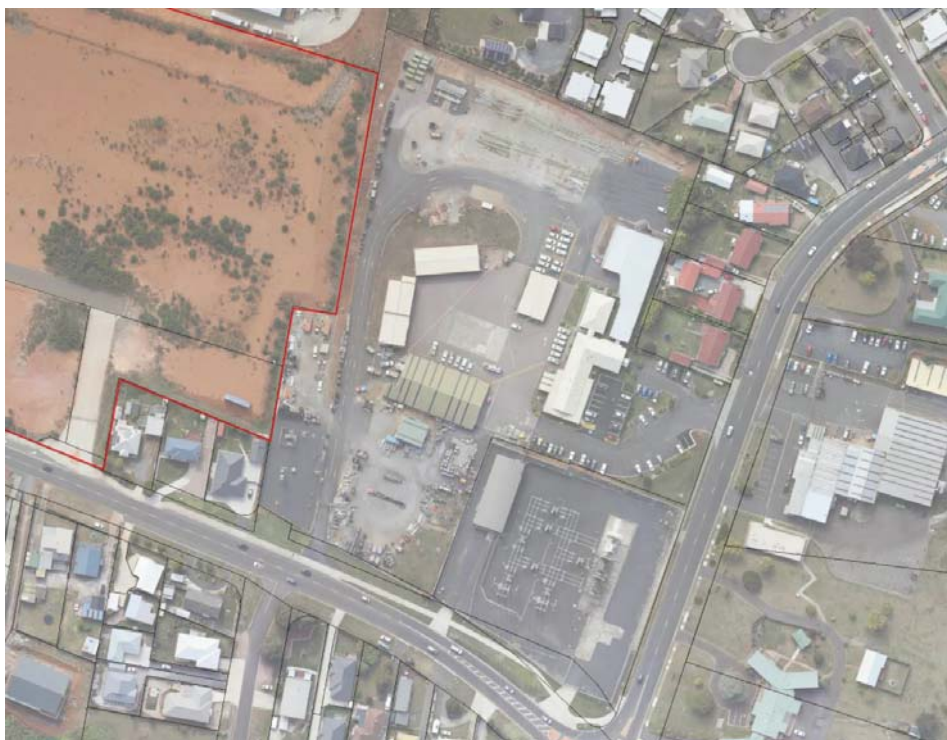
Figure 10 TasNetworks substation centre of image. Base image and data from theLIST ( www.thelist.tas.gov.au ) © State of Tasmania.
