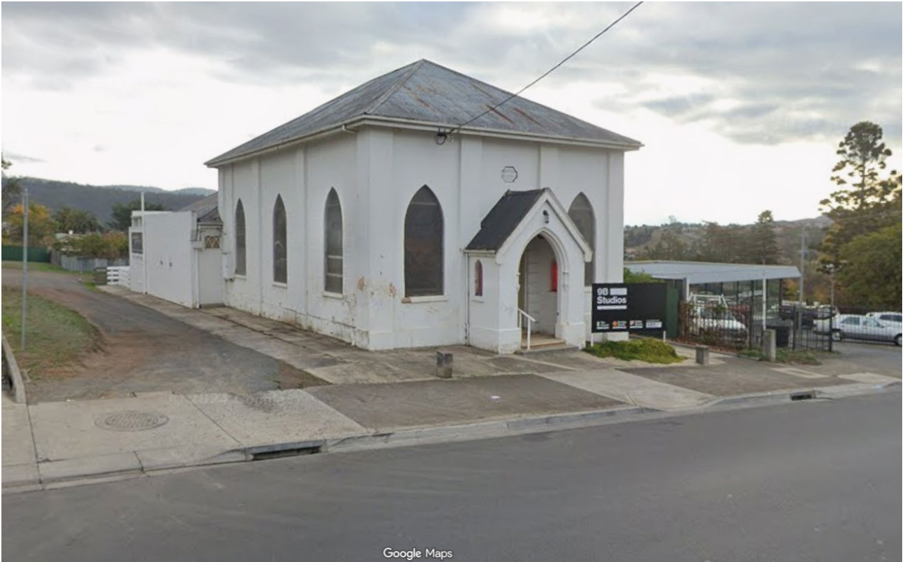
Figure 2 Image of the site as viewed from Burnett Street (Source: Google Maps, May 2024)
