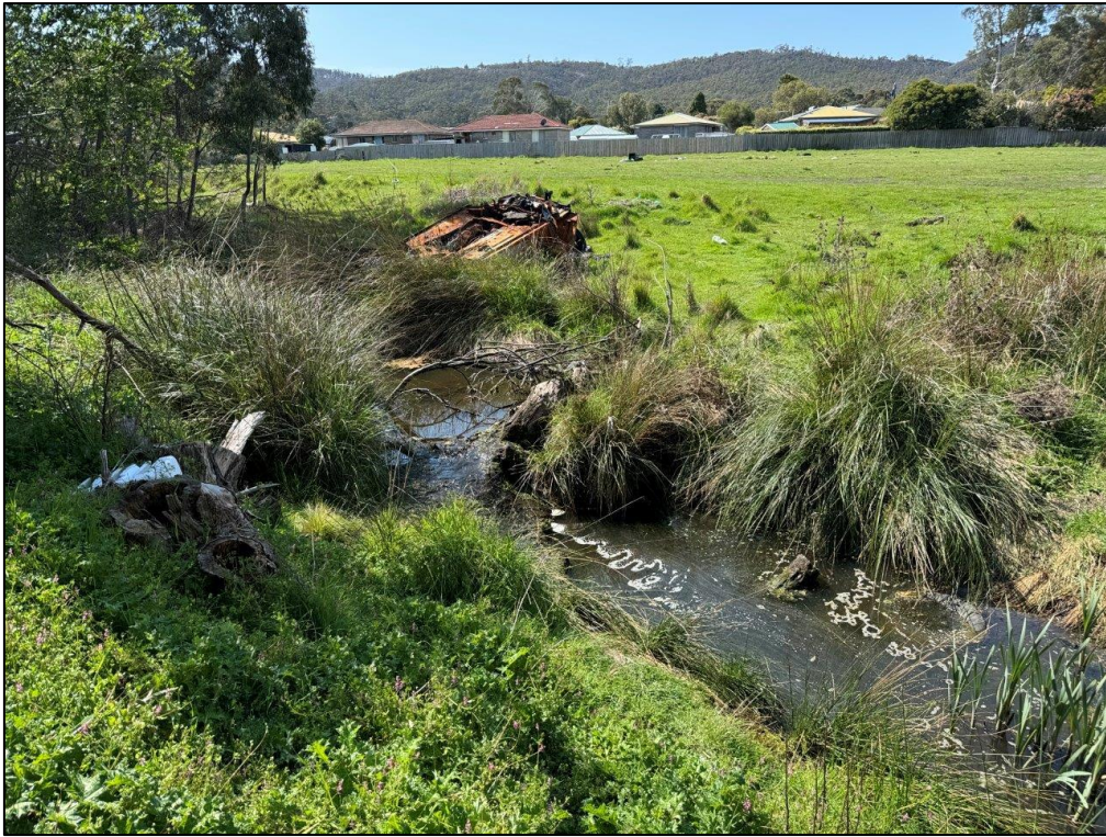
Plate 7. Degraded condition of Stokell Creek near Goodwins Road
