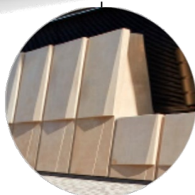
FT06 CONCRETE WALLS
